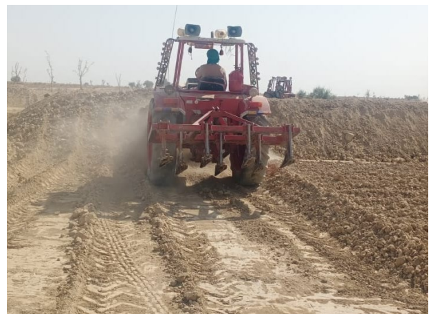
Figure 2: Embankment construction through the Joint Management Committee
