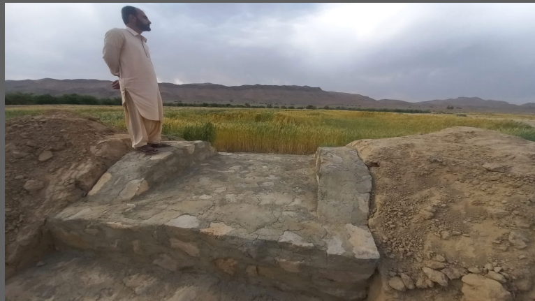
Overflow structure through: ADB Emergency Support Program
