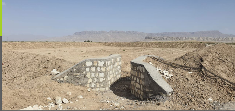
In and outflow structures
