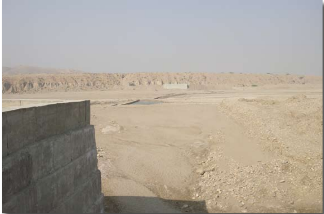
Figure 6. Low diversion weir between off-takes Sanghar
