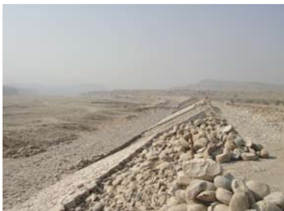
Figure 4. Embankment with stone pitching
