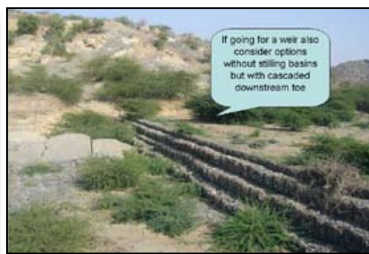
Figure 15. Weir with cascaded toe
