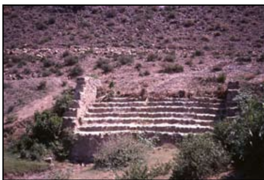
Figure 14. Stepped drop structure
