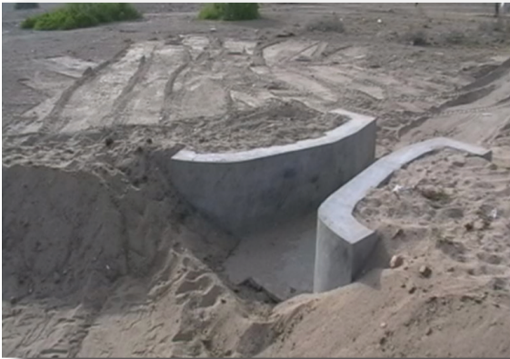
Controlled intake structure with gated intake
