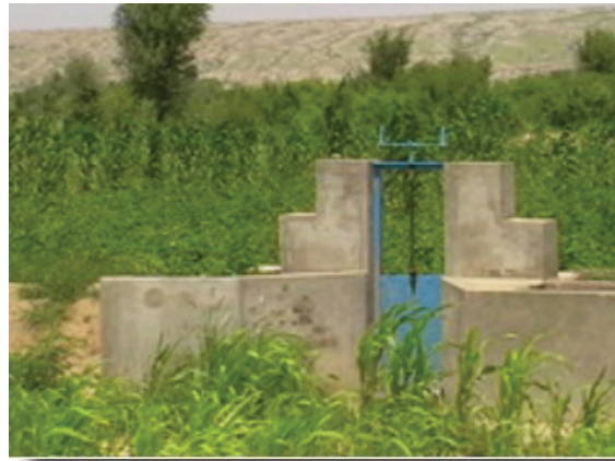
Controlled intake structure with gated intake
