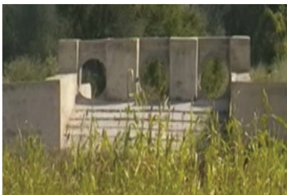
Spillway with stepped structure to break the force of water.
