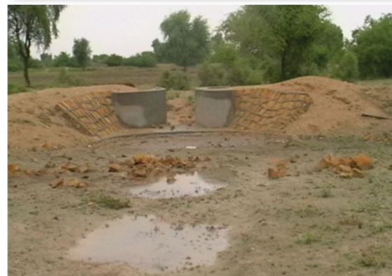
Constructing controlled intake: construction, back filling with soil and in operation (preferred design in EFAP)
