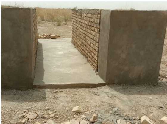
Controlled intake structure with stop log
