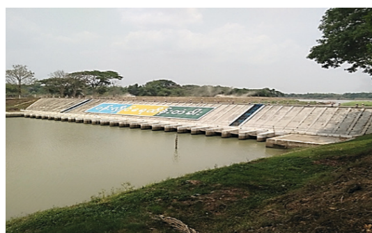
Figure (3) Downstream Side of the Pan Hlaing Sluice
