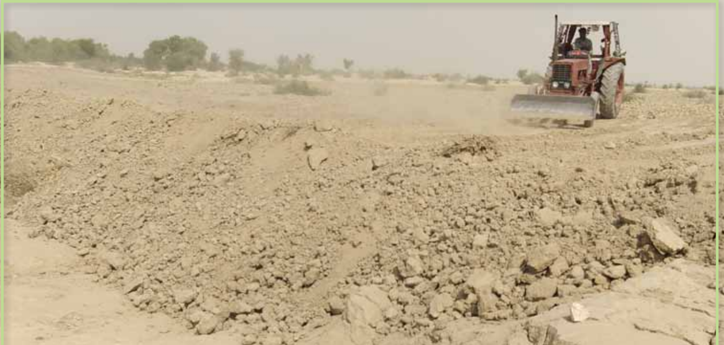
Land preparation in Nai Gaj spate system, constructing diversion structures and field bunds.
