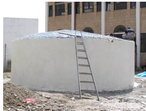
Construction 50 m 3 Ferro-Cement Tank, Ikhwan Thabit School
