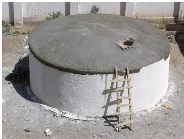
Construction 50 m 3 Ferro-Cement Tank, Ikhwan Thabit School
