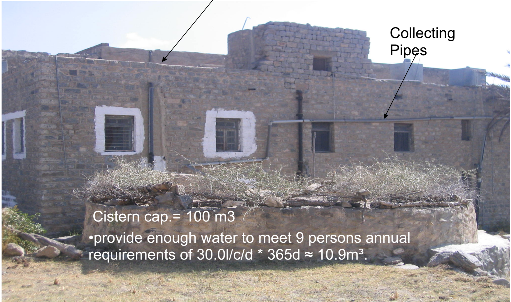
Roof rainwater Harvesting (Dr. Taha's house)
