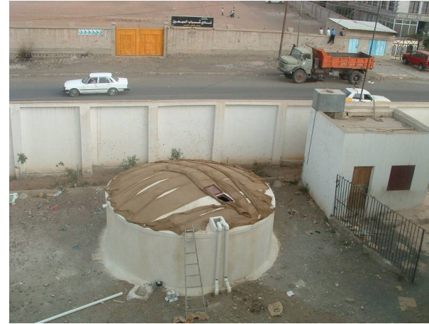
Construction 50 m 3 Ferro-Cement Tank, Ikhwan Thabit School
