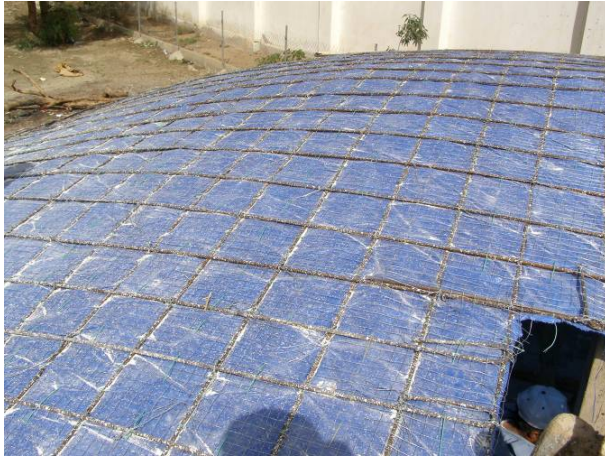
Construction 50 m 3 Ferro-Cement Tank, Ikhwan Thabit School
