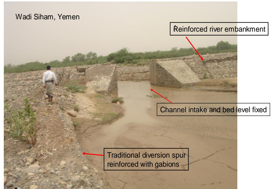
Improved flood channel open intake
