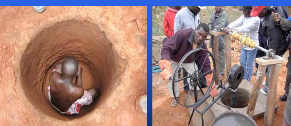
Well reducer rings Reducing the top diameter of a well to install a well cover and a pump
