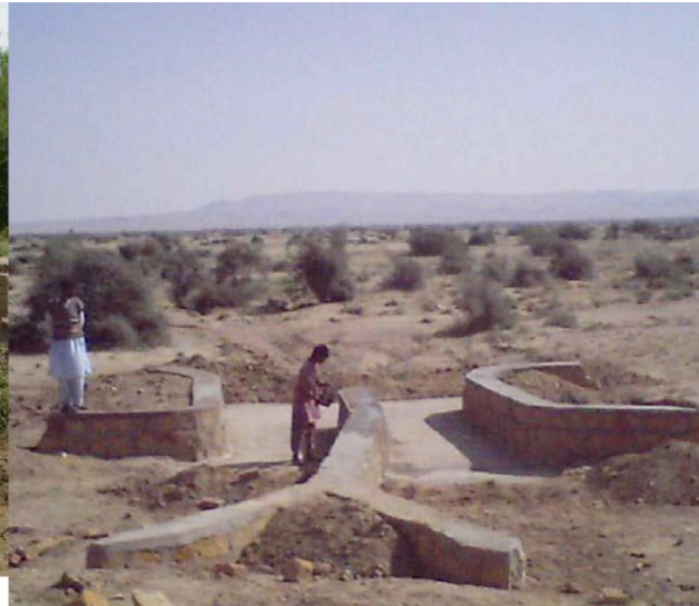
A low cost masonry stone work to divide spate flows – Designed and made by PARC in Dadu district.
