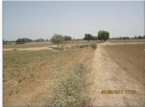
A traditional Free Intake from river to field made of soil – Jamshoro District
