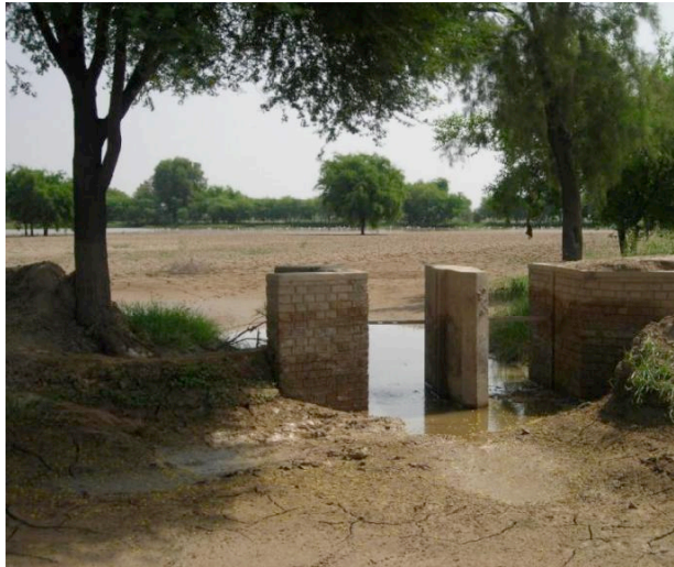
A traditional Free Intake from river to field made of soil – Jamshoro District
