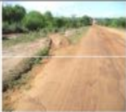
Rain water to be diverted into a ditch through diversion
