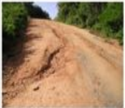
Erosion on the road if no water harvesting mechanism
