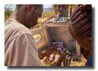
Figure 2: Connection of the moisture sensors to the board
