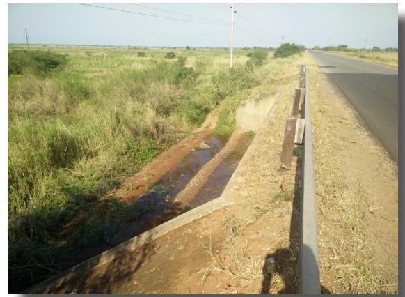
Figure 2: Bridge sill determining water level in upstream floodplain (Mozambique)
