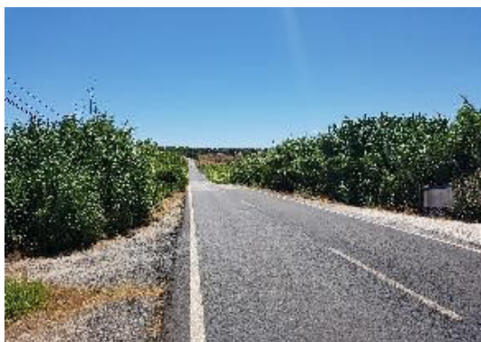
Figure 1: Floodway (Sado Plain, Portugal)
