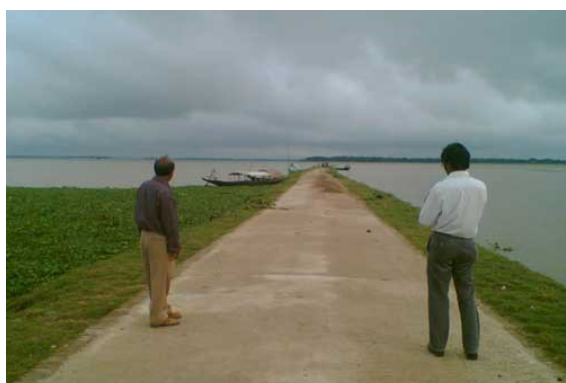
Figure 4: Submergible road in flood plain in Bangladesh ( http://www.lged.gov.bd/ )
