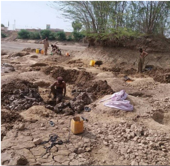
Figure 4: Seepage water collection from the dry reservoir May 2017
