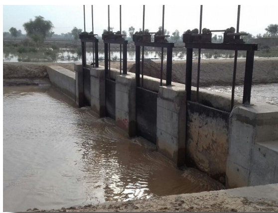
Figure 2: One of the water channels from Mini Barrage at Bhang
