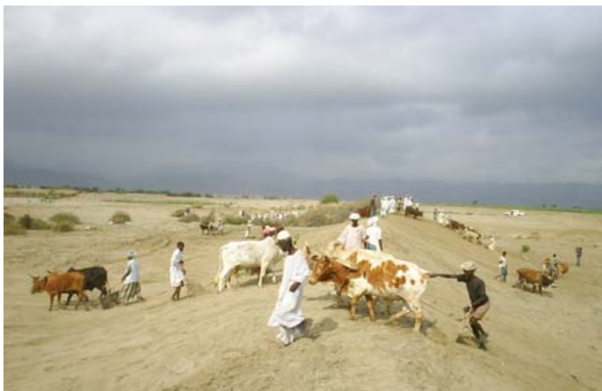
Figure 6: Traditional bund intake under construction using draught animals in Eritrea
