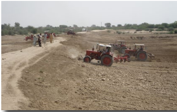
Figure 15: Earthen embankments under construction
