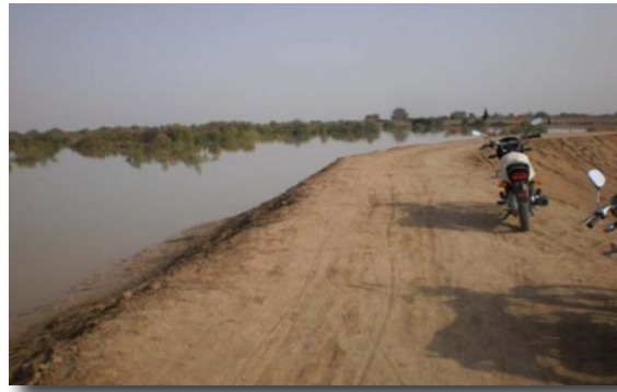
Figure 16: Earthen Embankment used for transport
