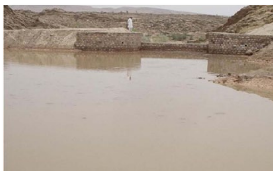
Figure 2: A low crest weir for water storage
