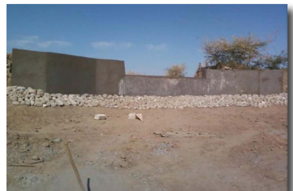
Figure 10: RCC spillway (Upstream) Kot Musa, DI Khan
