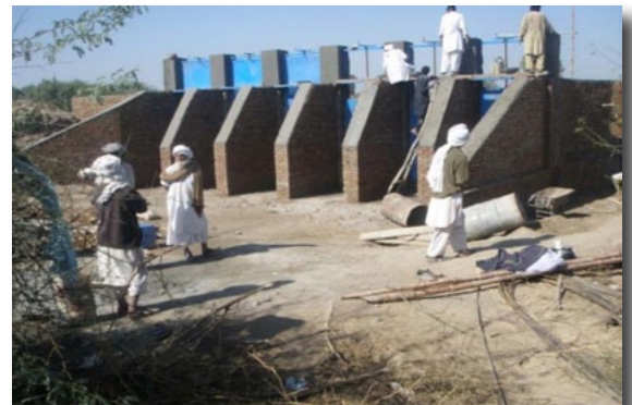
Figure 4: Gated Diversion Structures (1)
