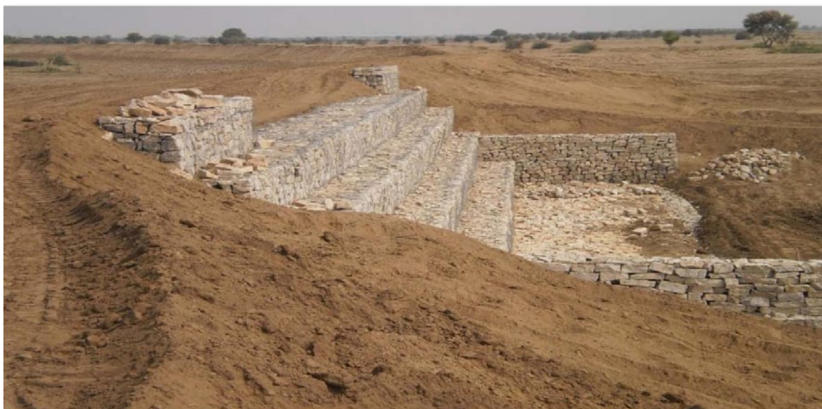
Figure 12: Stone Gabion Spillway, KPK (2)
