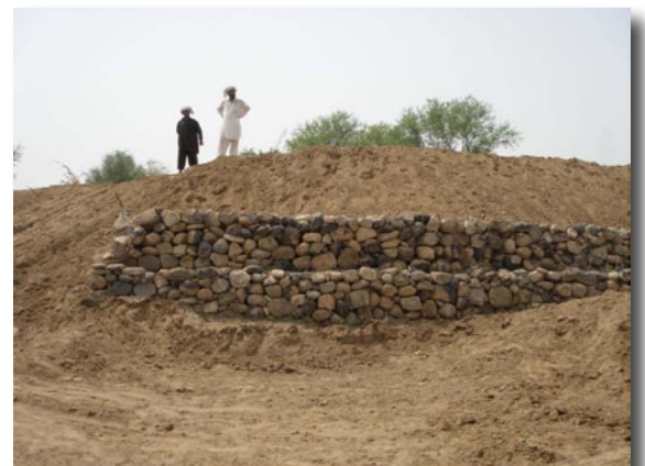
Figure 14: Retaining wall under construction
