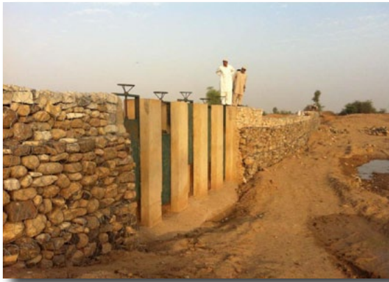
Figure 7: Gated Diversion Structures (2)
