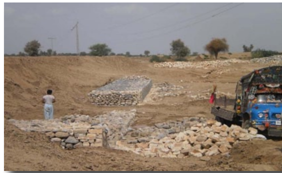
Figure 22: A bed stabilization weir
