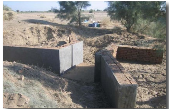
Figure 18: Field Inlet structure (under construction)
