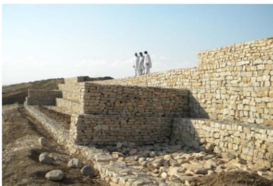
Figure 9: Stone Gabion Spillway, KPK (1)
