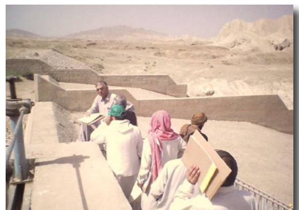
Figures 3 and 4. Gated and un-gated weir controlled off-stream water diversion to water tanks
