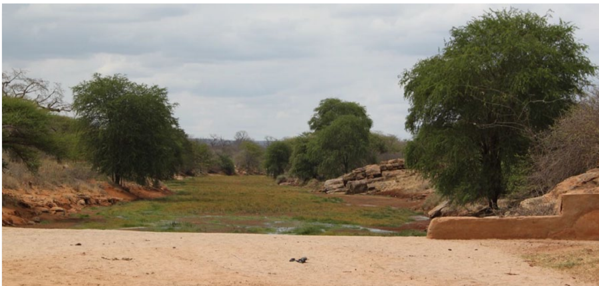
Figure 23. Downstream view of a sand dam in the Ilikoni Valley, Kenya.
