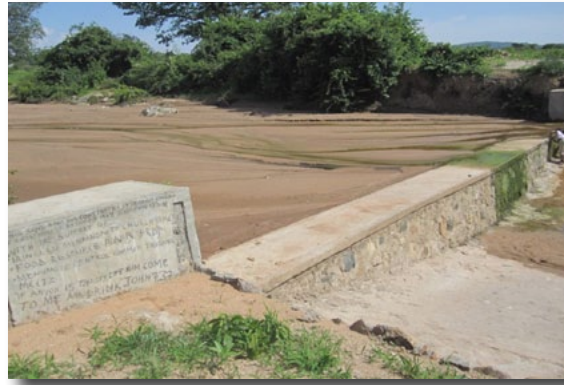
Figures 11 and 12. Stone masonry structure in the dry river bed for the sand dam
