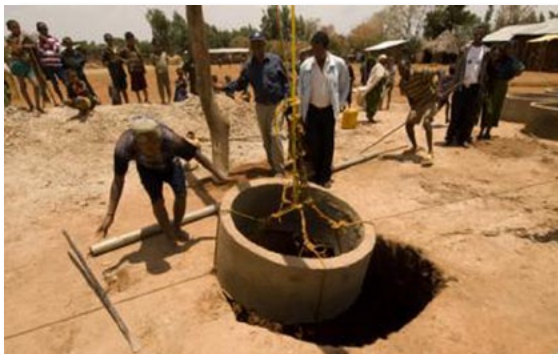
Figure 29. Construction of dugwell
