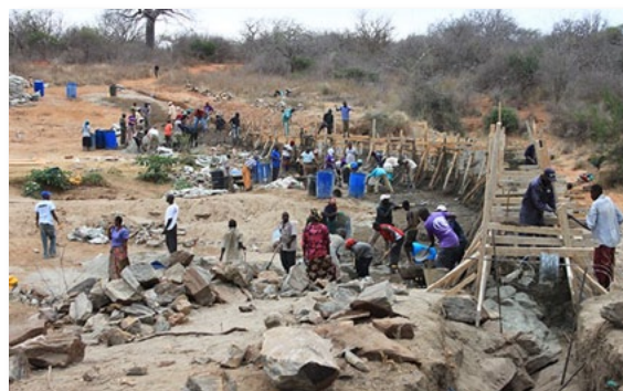
Figure 28. Dam under construction
