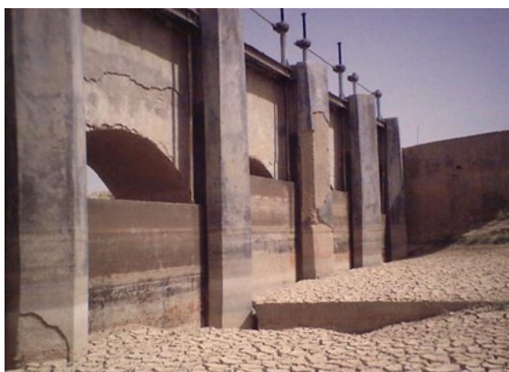
Figures 3 and 4. Gated and un-gated weir controlled off-stream water diversion to water tanks
