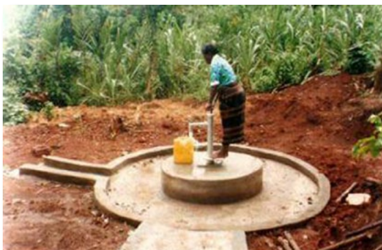
Figure 33. Protected dugwell in Uganda
