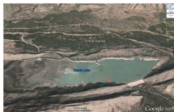
Figure 6. Tanda dam and command area
