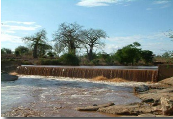
Figures 11 and 12. Stone masonry structure in the dry river bed for the sand dam
