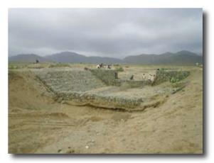
Figure 2. Flow division and channel bed stabilizer: important that apron has sufficient length
