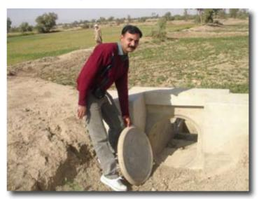
Figure 8. Improved field overflow structure
