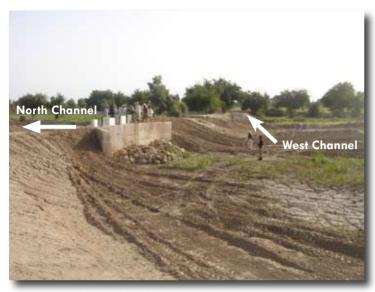
Figure 4. Solution: Flow division structure
