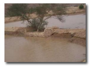
Figure 6. Stone reinforced overflow structure
