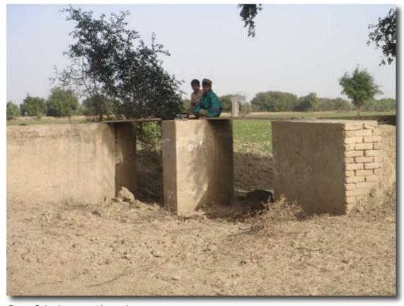
Figure 9. Intake gate with stop-logs
