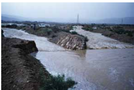
Figure 1: Traditional diversion structure, Yemen
