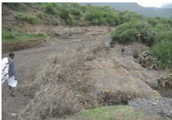
Figure 5: Ethiopia, after large flood: damaged gabion structure (left) (Kidane, 2009); huge gully formation (right)
