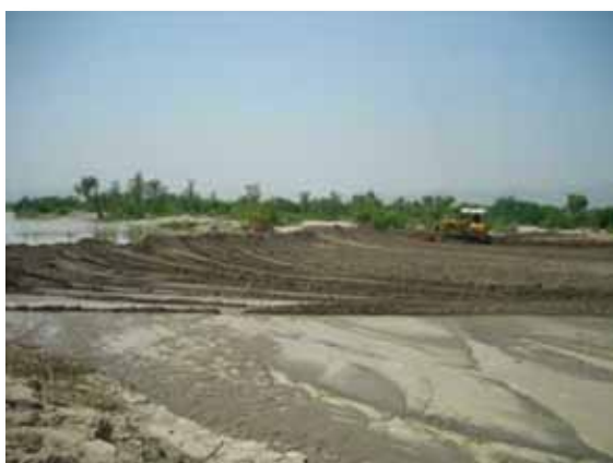
Figure 15: Field and canal bund maintenance using bulldozers in Pakistan.
