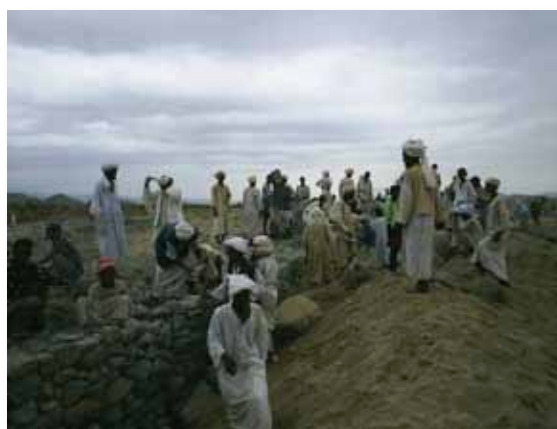
Figure 14: Re-enforcing traditional guide bunds with gabions, Wadi Labka, Eritrea
