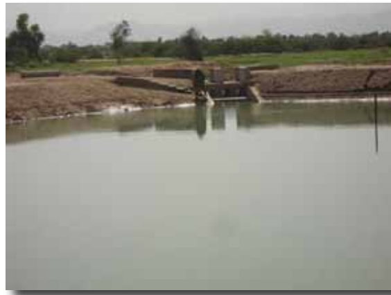
Figure 11: Renovated ponds for domestic and livestock water supply, Pakistan
