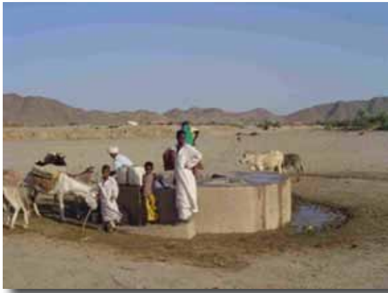
Figure 10: Improved well in river bed for domestic water supply, Eritrea
