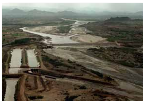
Figure 13: Modernized spate irrigation headwork with settling basin and breaching band, Yemen
