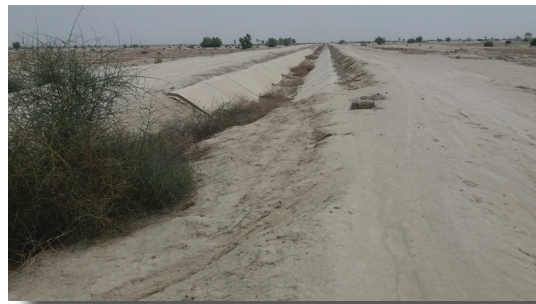
Figure 8 One of the Wahs that has been lined with concrete slabs
