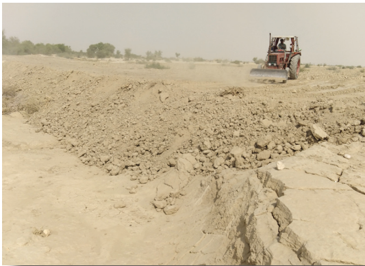
Figure 14 Ploughing and planing for moisture conservation
