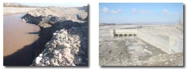
Fig 2: Bund and diversion structure in the Surkhrod ephemeral river and Amu basin area (MEW, 2012) Left: Traditional bund; Right: Modern diversion structure.
