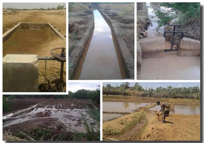
Figure 9: Images of different Spate irrigation projects using structures to take water from wadi's towards the fields.
