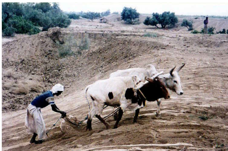
Figure 3.1 Bund construction using bullocks and scraper board Eritrea
