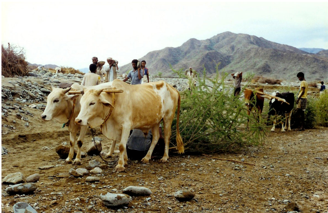
Figure 11.1 Collection of shrubs for the repair of flood diversion spurs, Eritrea
