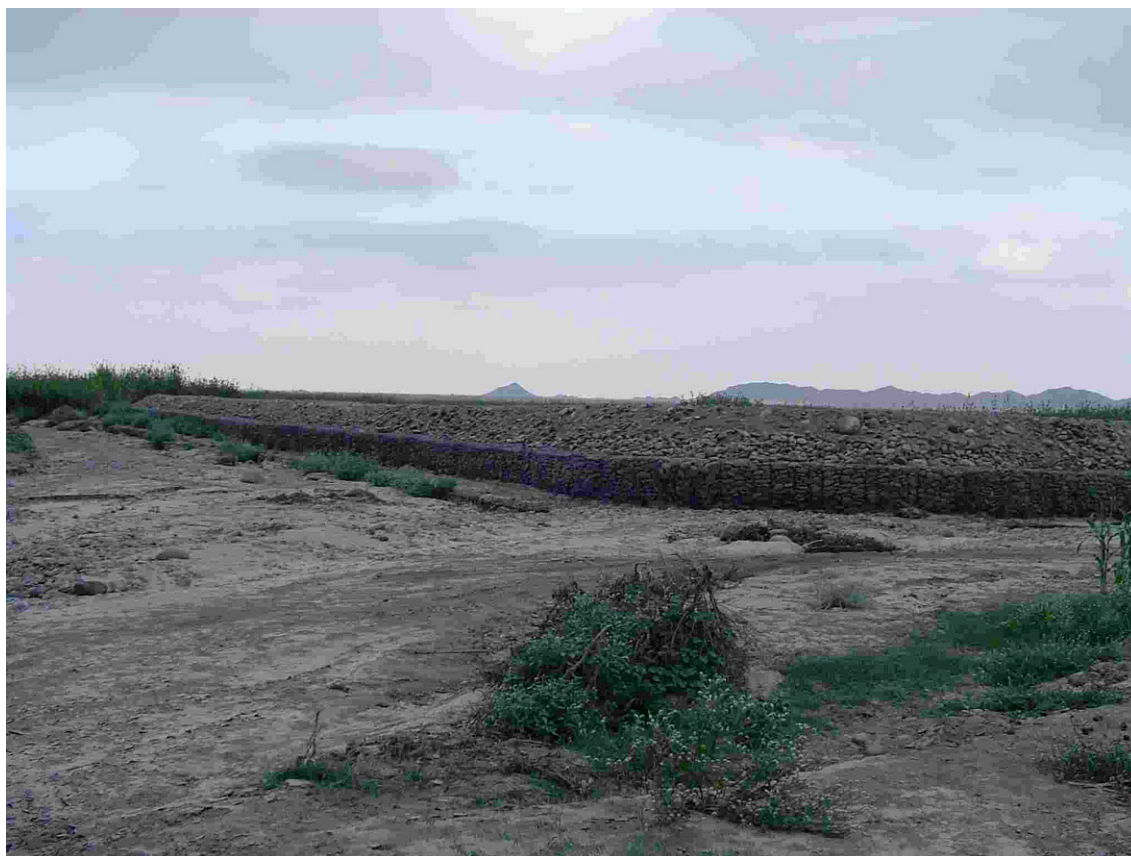
Figure 10.27 Gabion flow bifurcation structure in Eritrea
