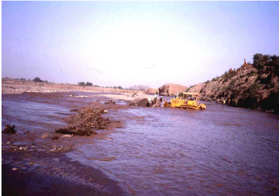
Figure 10.11 Bulldozer repairing a traditional diversion spur during a flood recession - Wadi Rima in the Yemen in the mid 1980s
