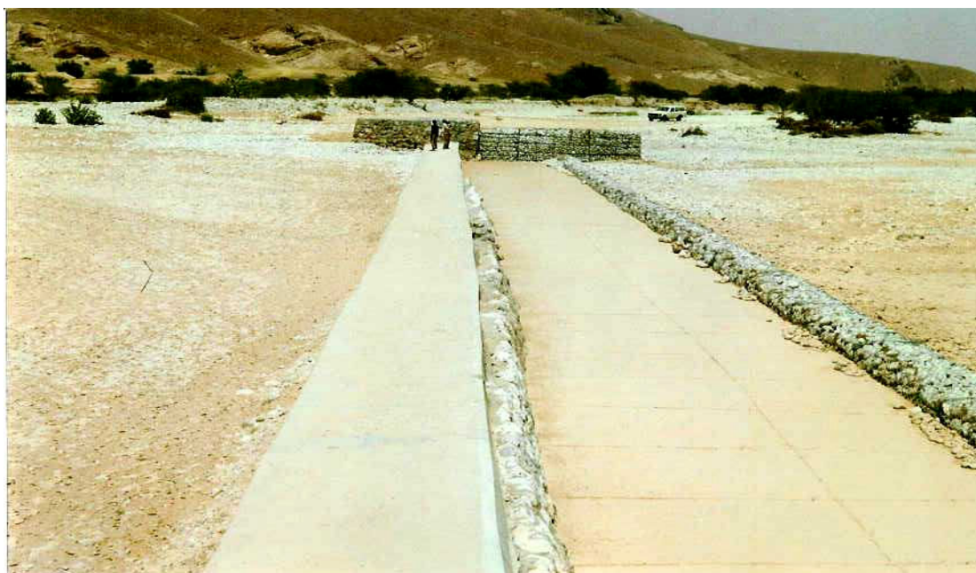
Figure 10.10 Rehabilitated traditional weir in Wadi Haudramat
