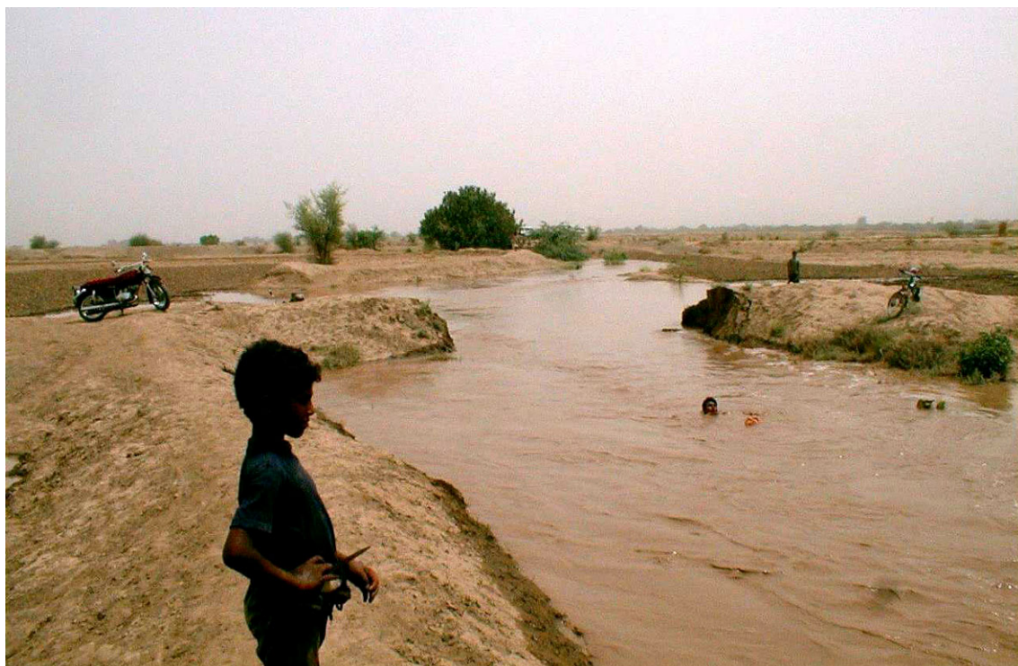
Figure 10.24 Breached canal diversion bund, Wadi Zabid, Yemen in 2003
