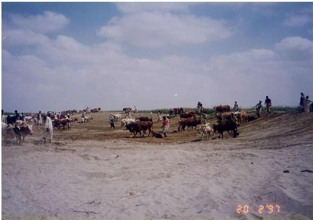
Figure 10.6 Bund construction with bullocks and scraper boards, Eritrea
