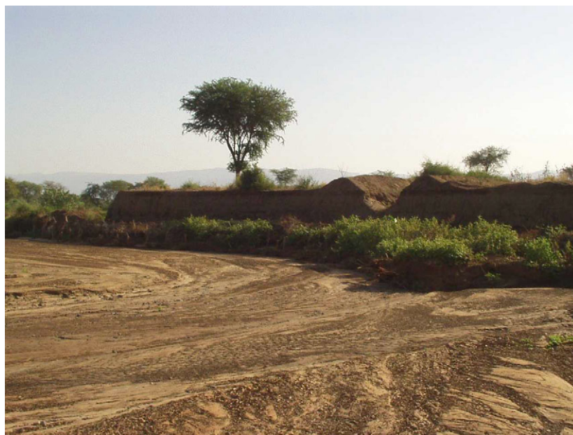
Figure 11.2 Canal head abandoned due to lowering of the riverbed and erosion of the riverbanks, Yandefero, Ethiopia
