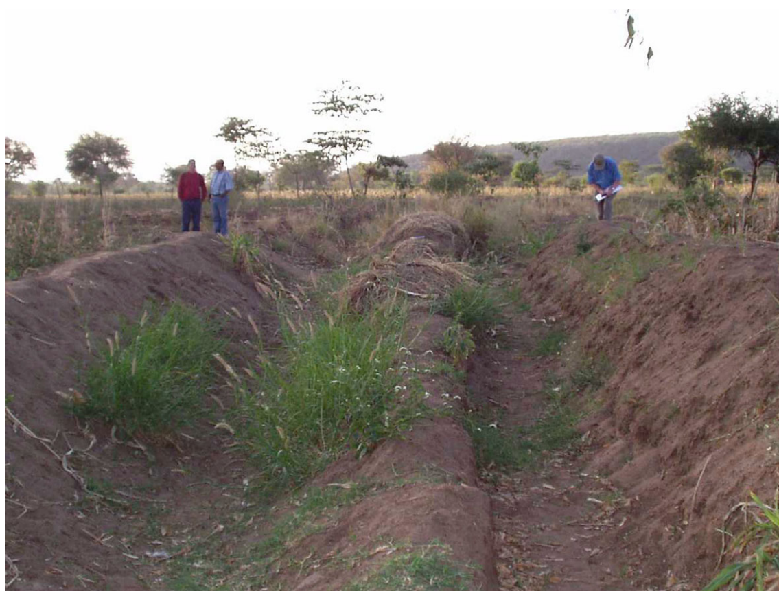
Figure 7.1 Flow division in a flood canal, Yandafaro, Ethiopia
