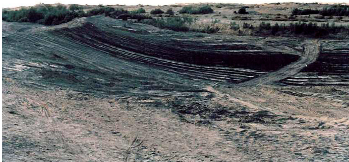
Figure 8.3 Earthen diversion bund (ghanda) constructed by bulldozer, Pakistan
