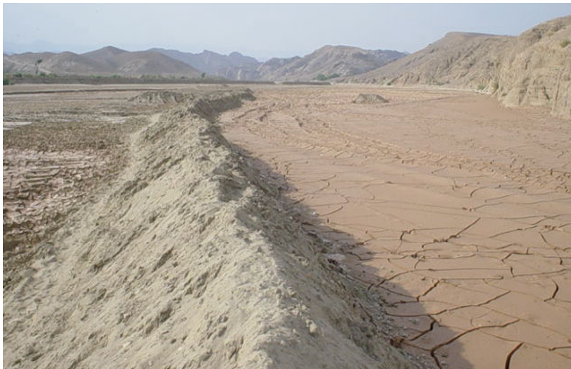
Figure 10.4 Traditional spate irrigation intake in Pakistan
