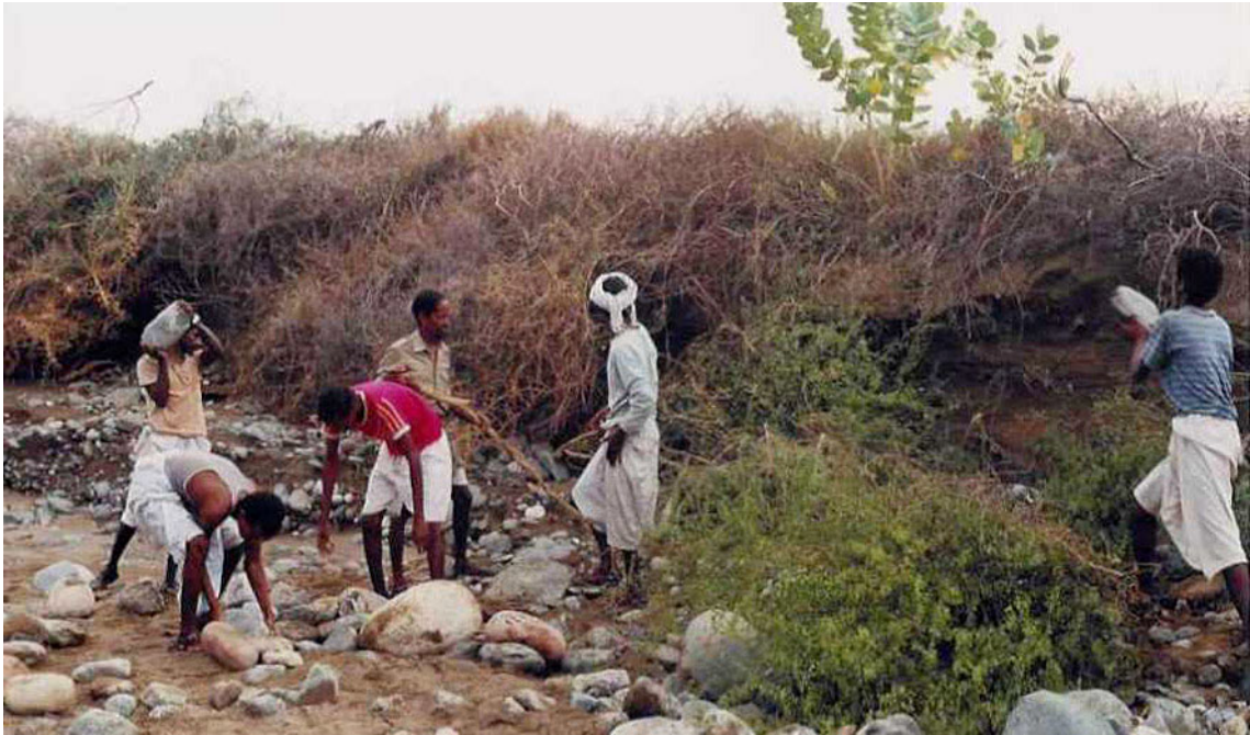
Figure 10.19 Bank protection using brushwood and boulders – Wadi Laba Eritrea
