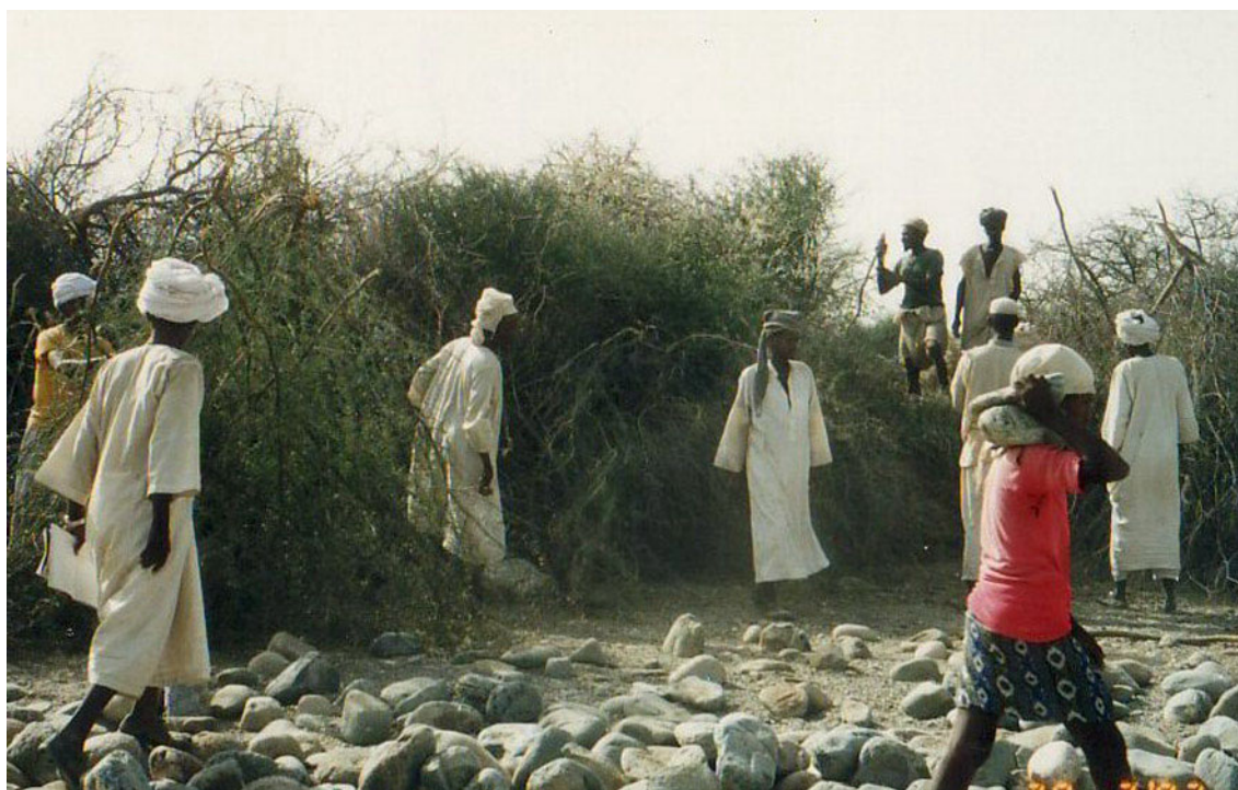
Figure 3.3 Brushwood being used to protect the banks of spate canal, Eritrea
