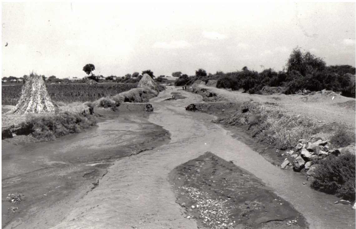
Figure 10.23 Breached canal diversion bund, Wadi Zabid, Yemen in 1980
