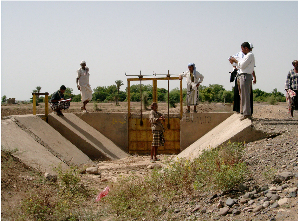
Figure 10.26 Gated combined check/drop structure – Yemen
