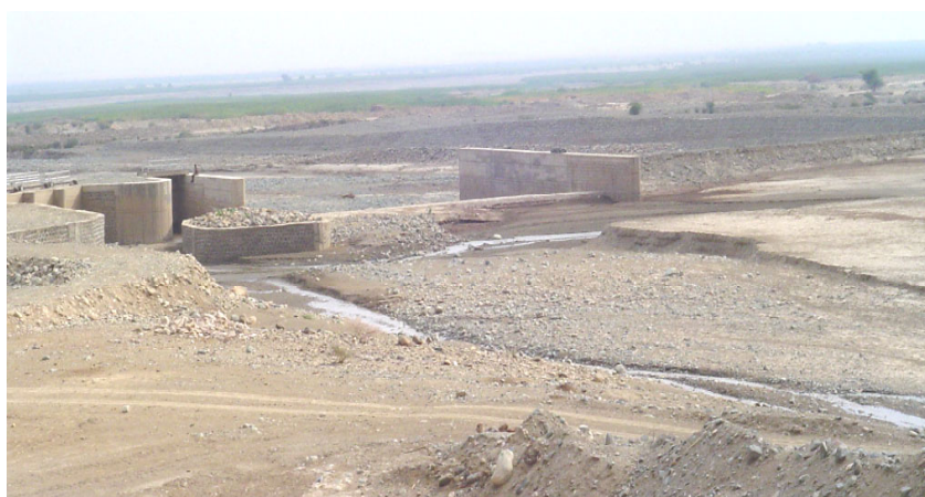
Figure 10.16 Spate diversion structure constructed at Wadi Laba, Eritrea
