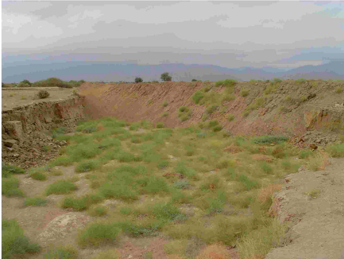
Figure 8.4 Bund constructed by bulldozer plugging a gully in the irrigated area formed by earlier uncontrolled flooding
