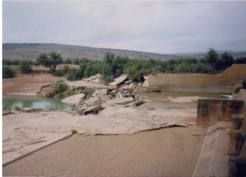
Figure 7.6 Diversion weir where part of the crest was blown-up by farmers as it interfered with the base flows, Pakistan
