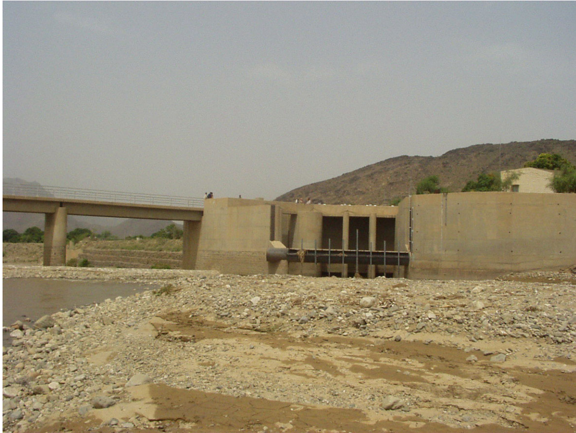
Figure 10.15 Trash deflector, Wadi Rima intake Yemen (2003)
