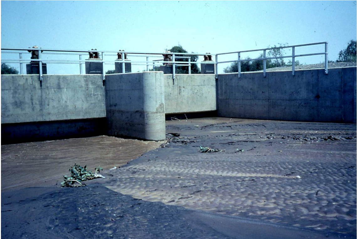
Figure 2.1 Heavily silted canal off take in a newly modernised spate scheme
