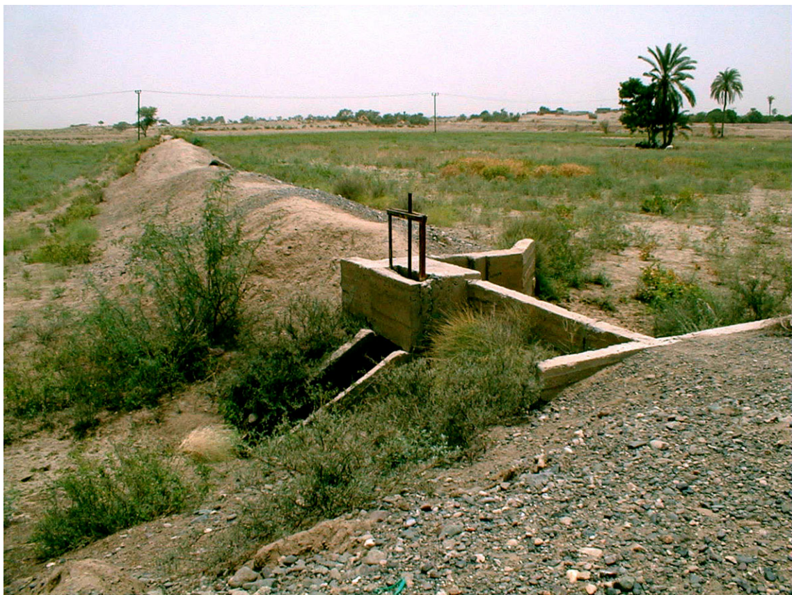
Figure 10.28 Gated field distribution and drop structure, Yemen
