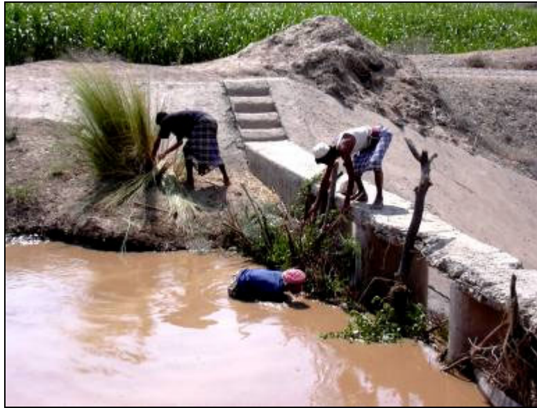
Figure 8.6 Farmers using brushwood to head up the flow in a canal in a modernized system, Wadi Tuban, Yemen
