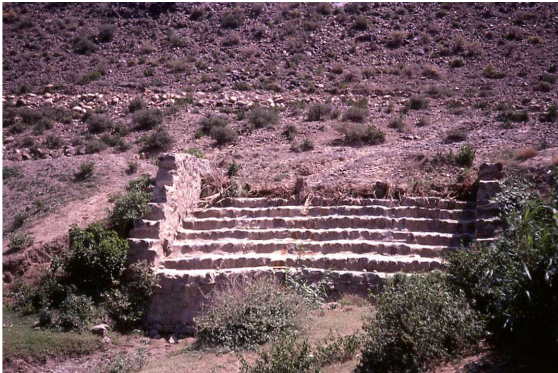
Figure 10.12 Side spillway constructed by farmers, Wadi Rima Yemen
