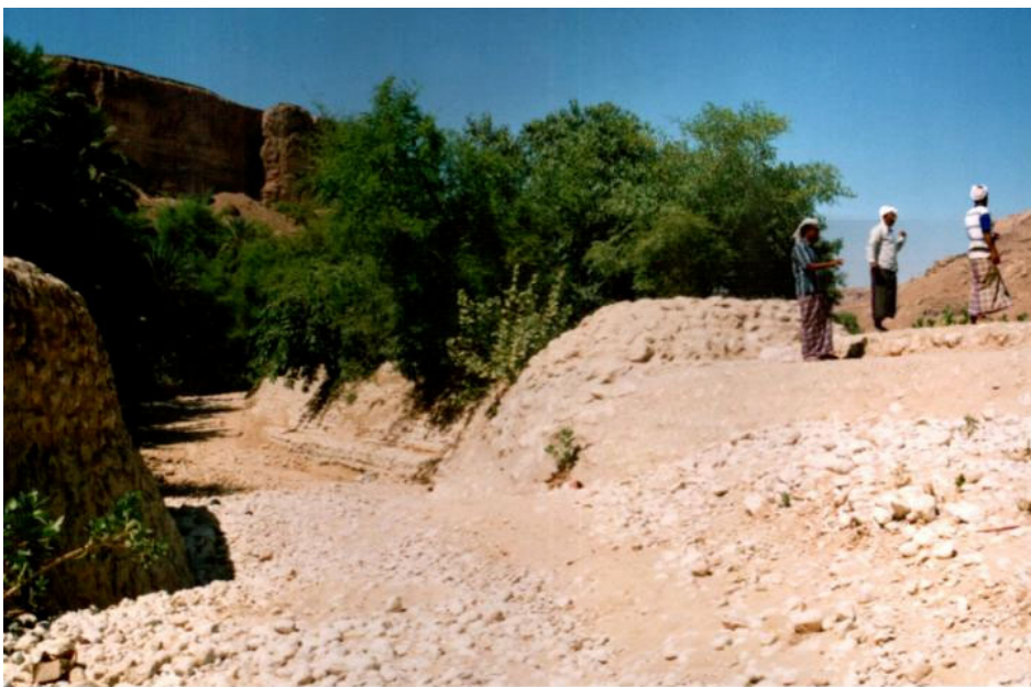
Figure 10.9 Canal head with Algamas forming the left and right sides of the canal entrance
