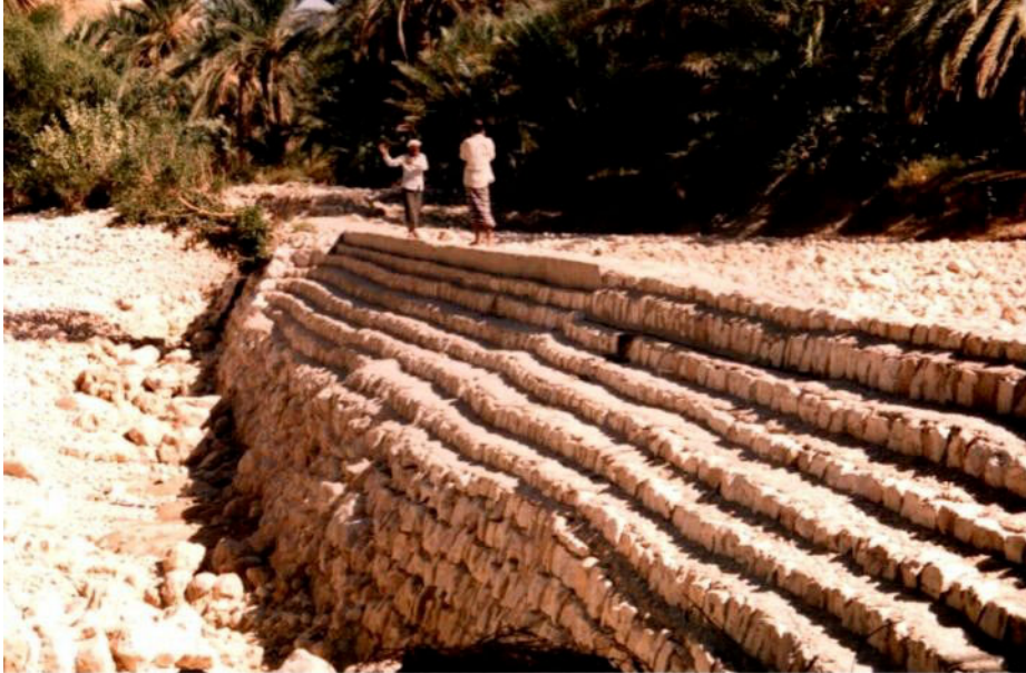
Figure 10.8 Diversion Weir with a stepped downstream face
