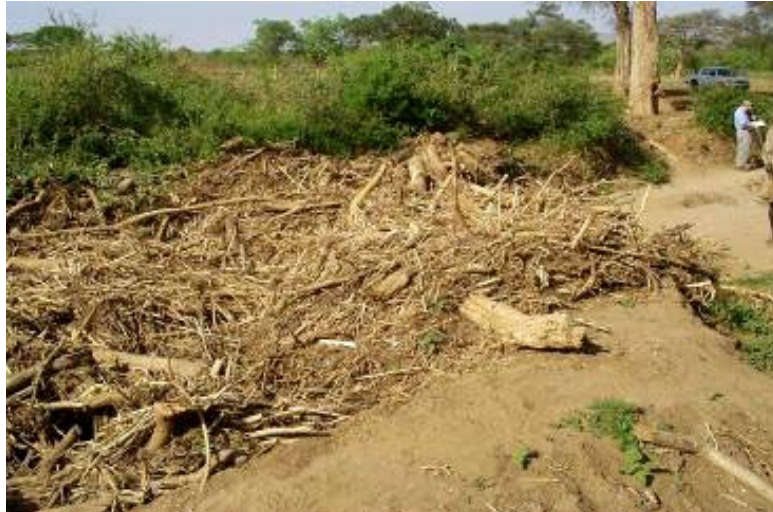
Figure A4.1 Trash completely blocking a small new intake located on the outside of an excessively sharp ( >90^\circ ) river bend in Ethiopia
