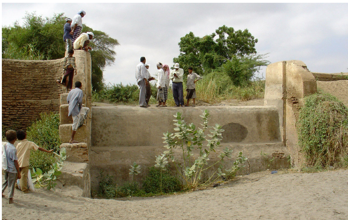
Figure 10.25 Traditional drop structure, Wadi Zabid, Yemen
