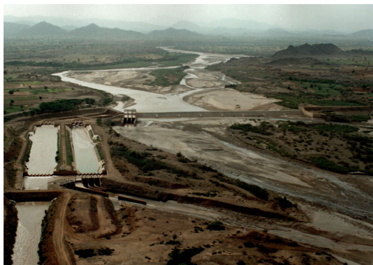
Figure 2.2 Wadi Mawr spate irrigation intake, Yemen
