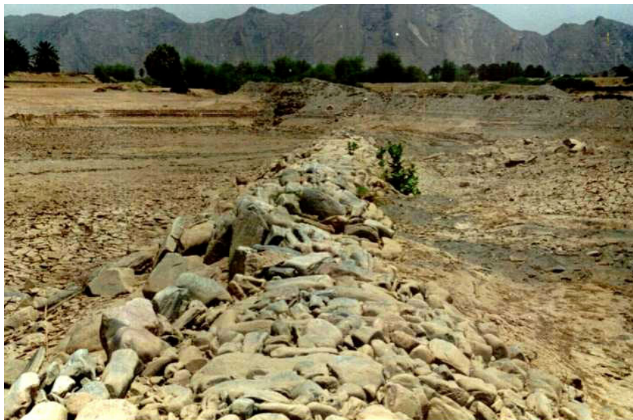
Figure 10.7 Partially breached diversion spur in Wadi Beihan, photographed from the wadi, looking towards the canal intake
