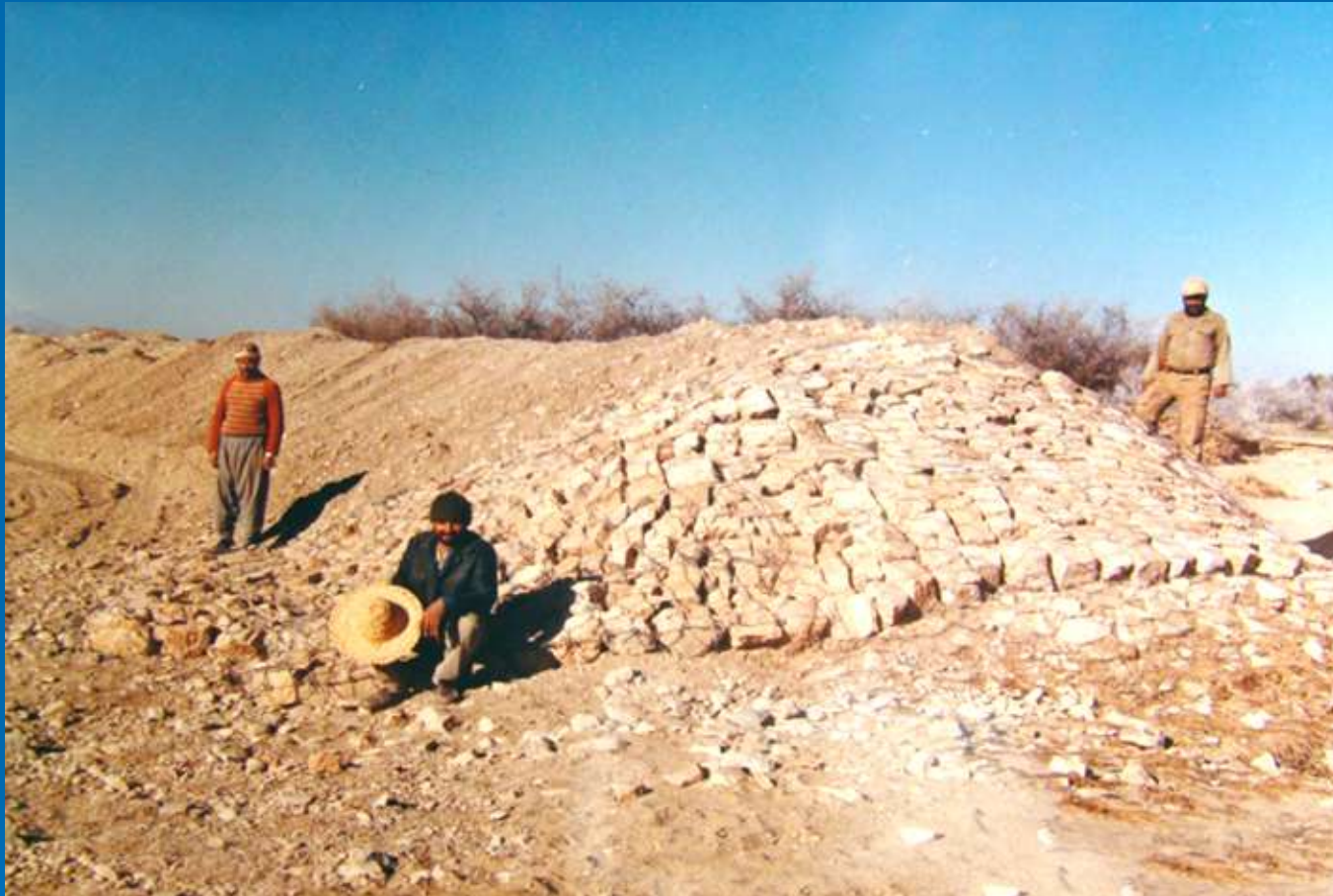
Fig. 17. A gabion mattress connected to a gabion apron protects the lower bank of an inundation canal in the Gareh Bygone Plain.
