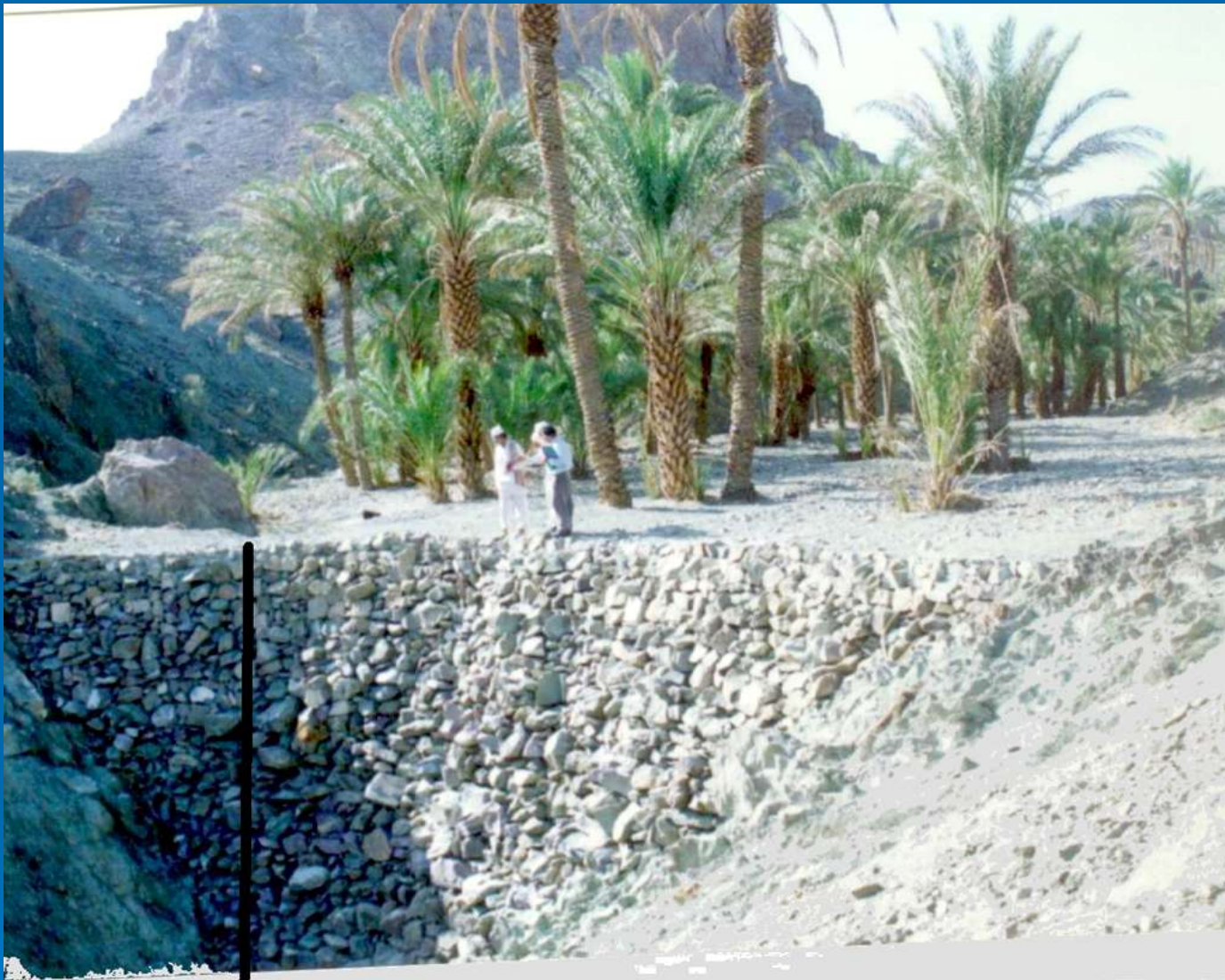
Fig. 7. Darband , a spate irrigation system in Baluchestān, SE Iran.
