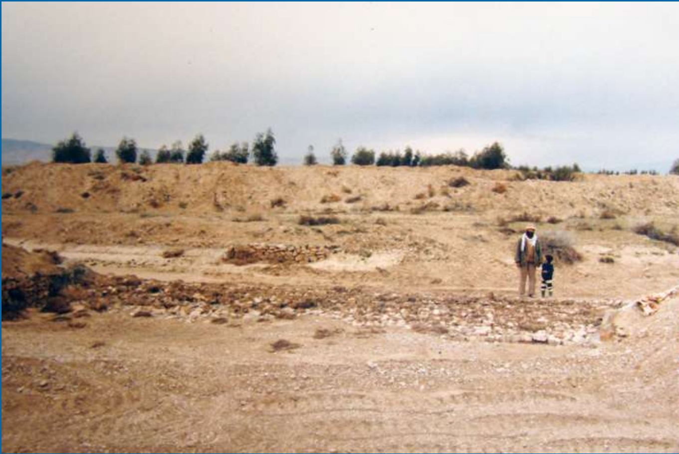
Fig. 14. A downstream view of a gabion apron with a triangular cross section. This apron is functioning well since its construction in 1984. The crest of this apron was raised 30 cm in 2002 after sedimentation raised the level of a sedimentation basin by about 20 cm.
