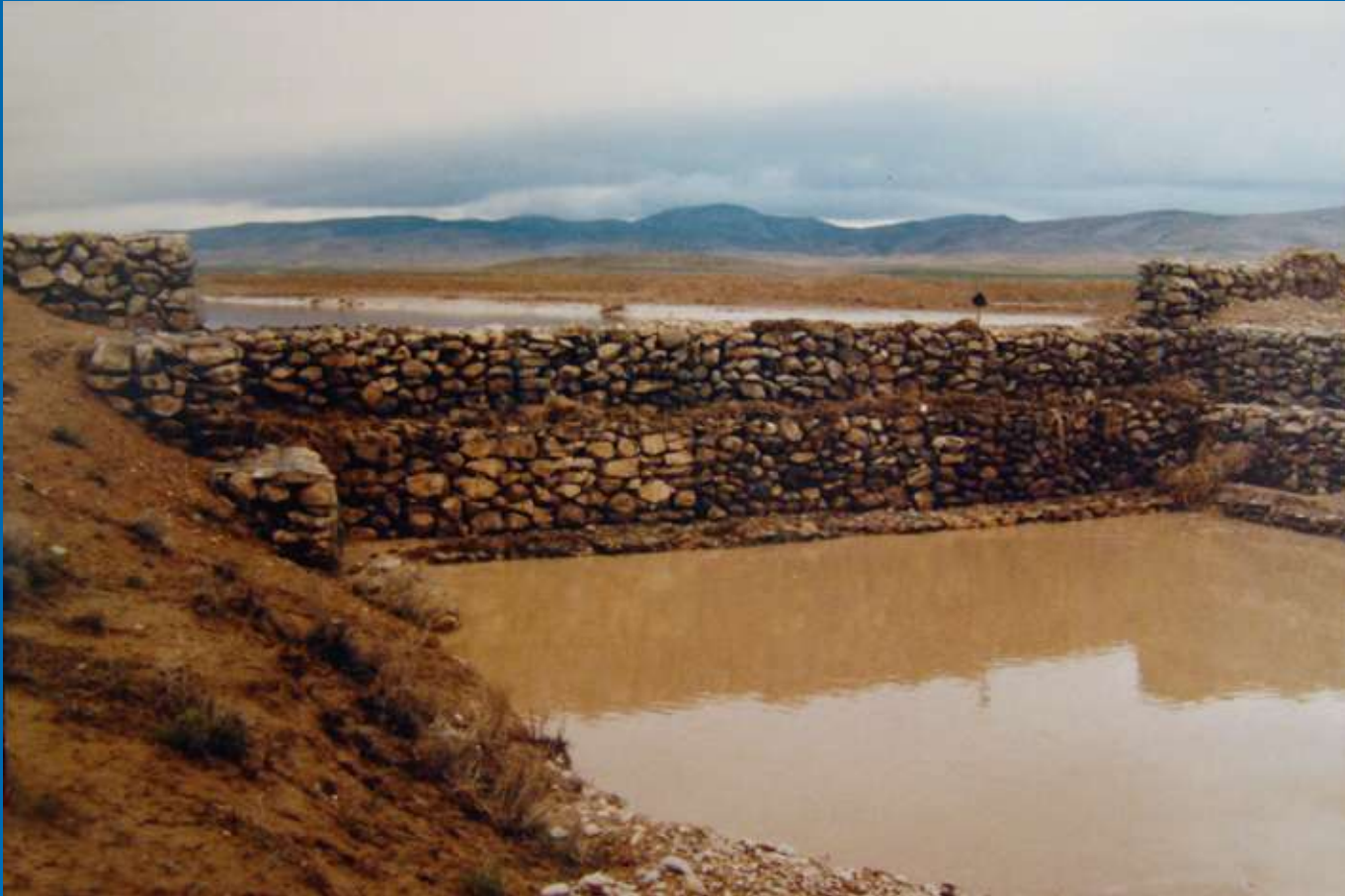
Fig. 21. A 3-row gabion weir at the Gooyom spate irrigation system. This weir diverted floodwater for irrigating 250 ha of wheat.
