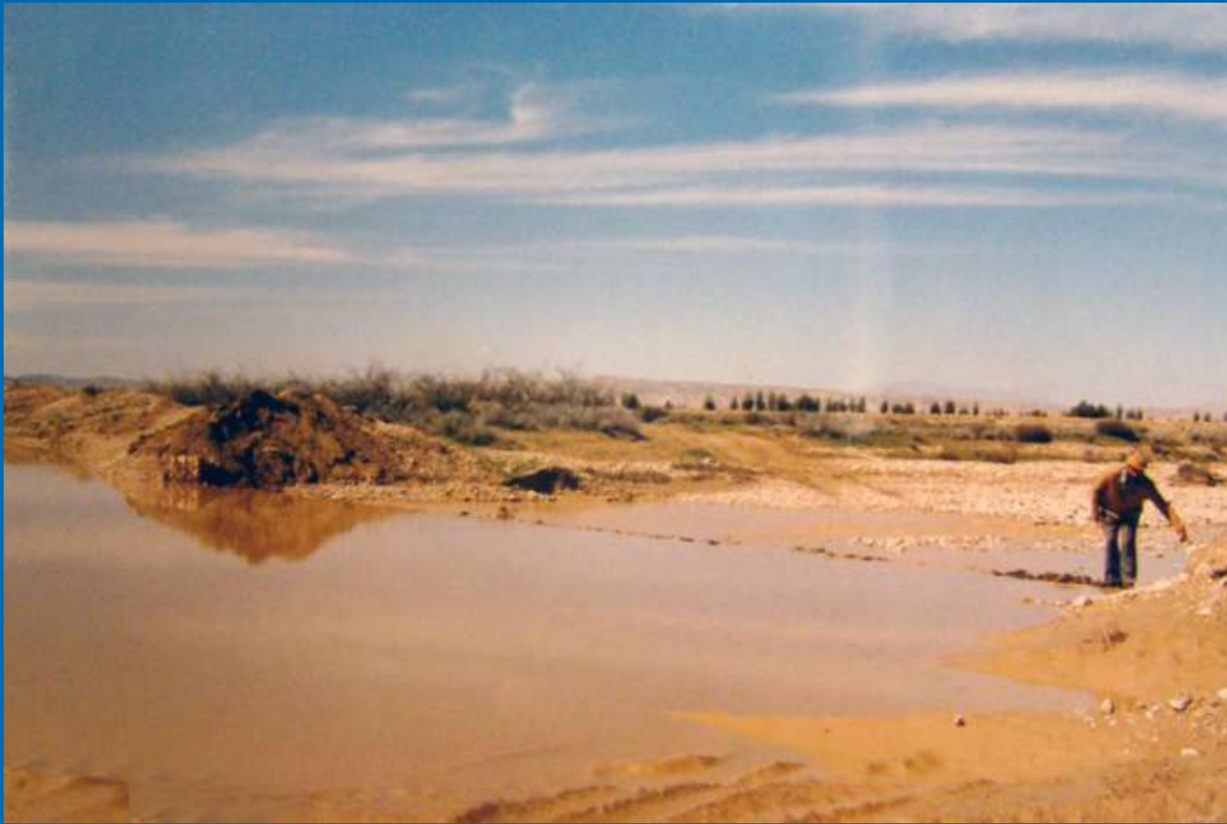
Fig. 15. The late Haj Mohammad Pashali is pointing to the water mark of the flood peak. This structure diverts floodwater for a 25 ha artificial recharge of groundwater system in the Gareh Bygone Plain.
