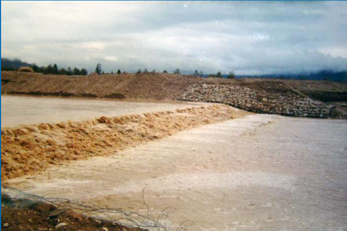
Fig. 16. A gabion apron with a triangular cross section in operation. A ski jump dissipates most of the kinetic energy of the flowing water.
