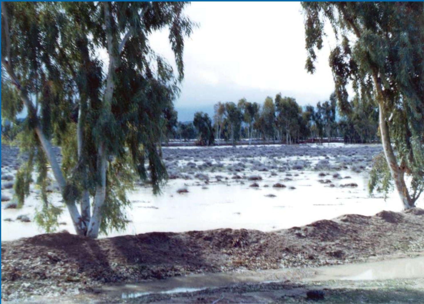
Fig. 12. Floodwater spreading for the artificial recharge of groundwater, Kowsar Station, Gareh Bygone Plain, SE Iran.
