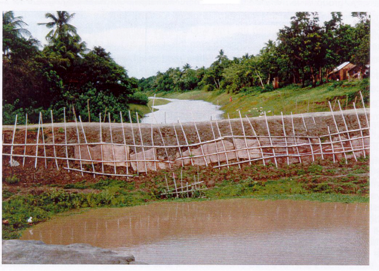
A Cross Dam Erected in a Khal (Royal Haskoning)
