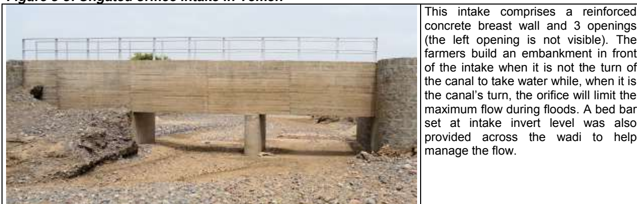
Figure 8-8: Ungated orifice intake in Yemen
