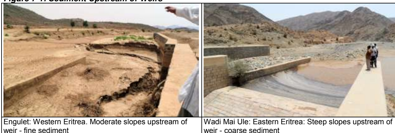
Figure 7-1: Sediment Upstream of Weirs
