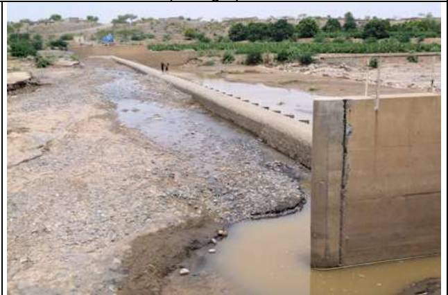
The divide wall has been cut back and enables flush of sediment upstream of the weir.
