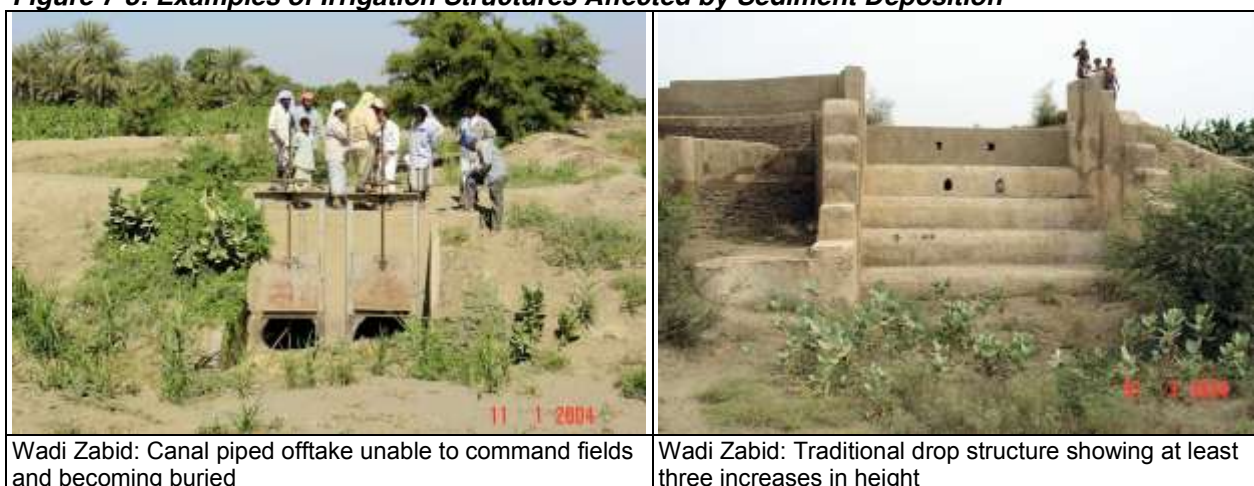
Figure 7-8: Examples of Irrigation Structures Affected by Sediment Deposition
