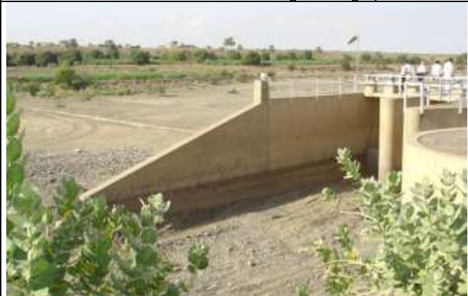
Wadi Zabid weir prior to cutting back of divide wall. Sediment upstream of weir has accumulated to weir crest level
