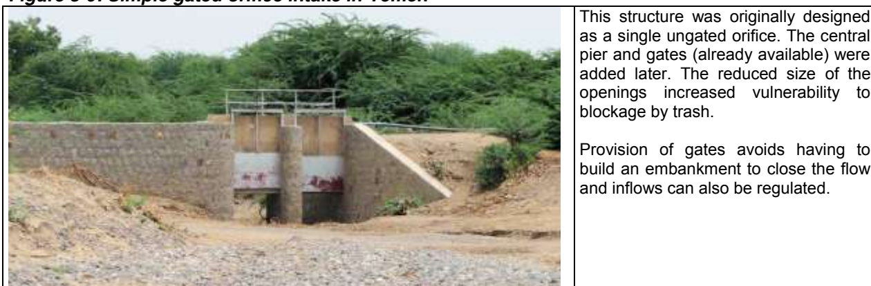
Figure 8-9: Simple gated orifice intake in Yemen
