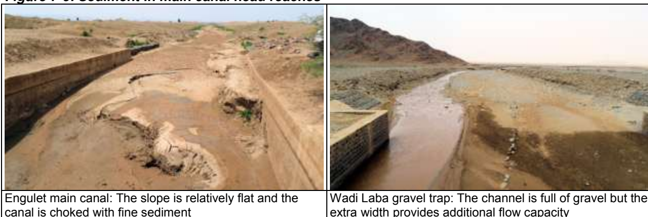
Figure 7-6: Sediment in main canal head reaches
