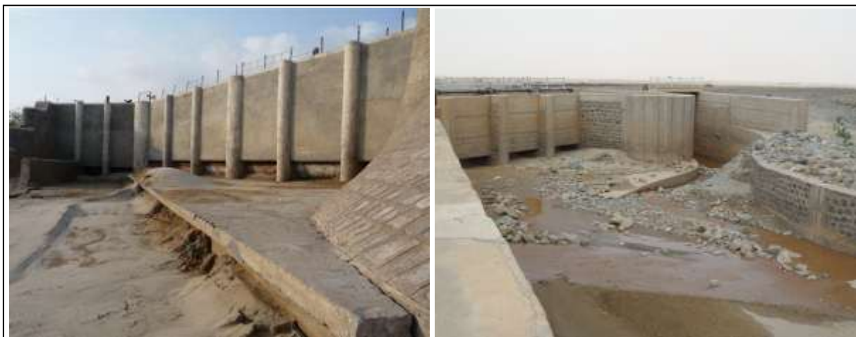
Figure 7-11: Typical Layout of Curved Channel Excluder
