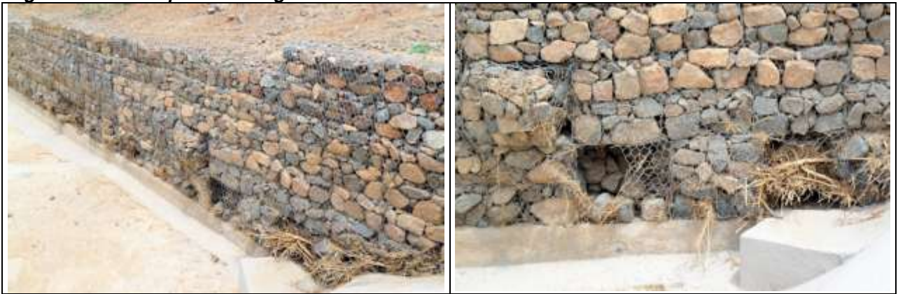
Figure 11-1: Example of Damage to Gabion Wall
