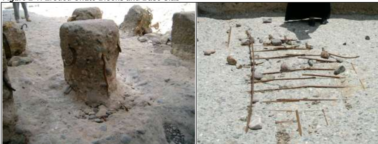
Figure 2-1: Eroded Chute Blocks and Base Slab
