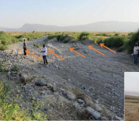
Complete utilization of diverted flood by gradually dissipating its energy through a series of distribution canals
