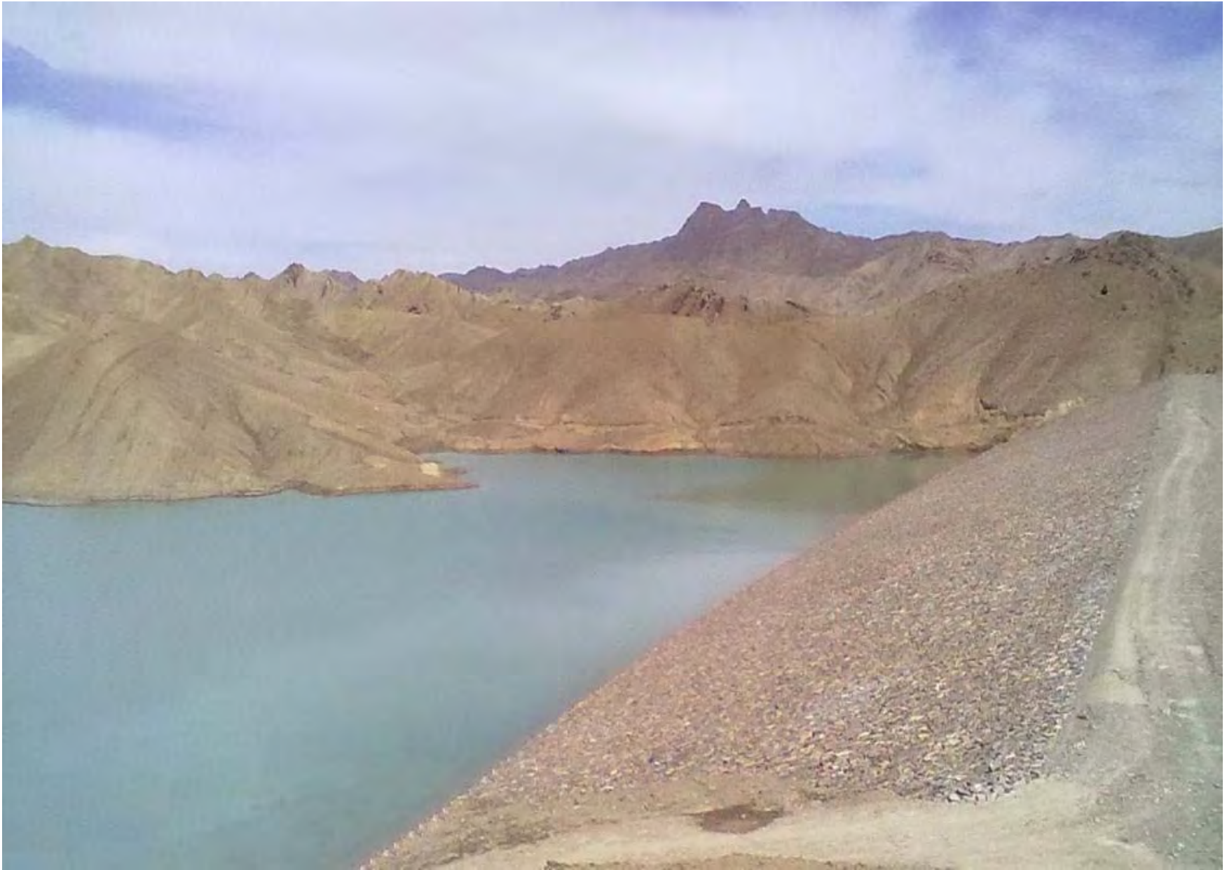
Arambi Dam – Embankment
