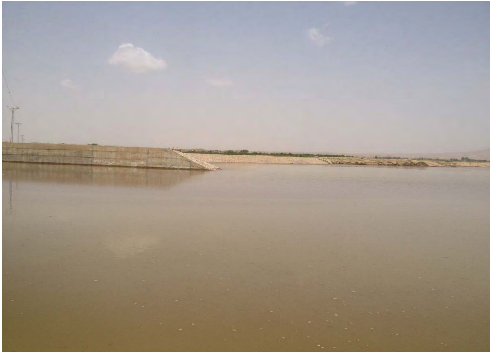
Bostan Dam – Distirct Pishin
