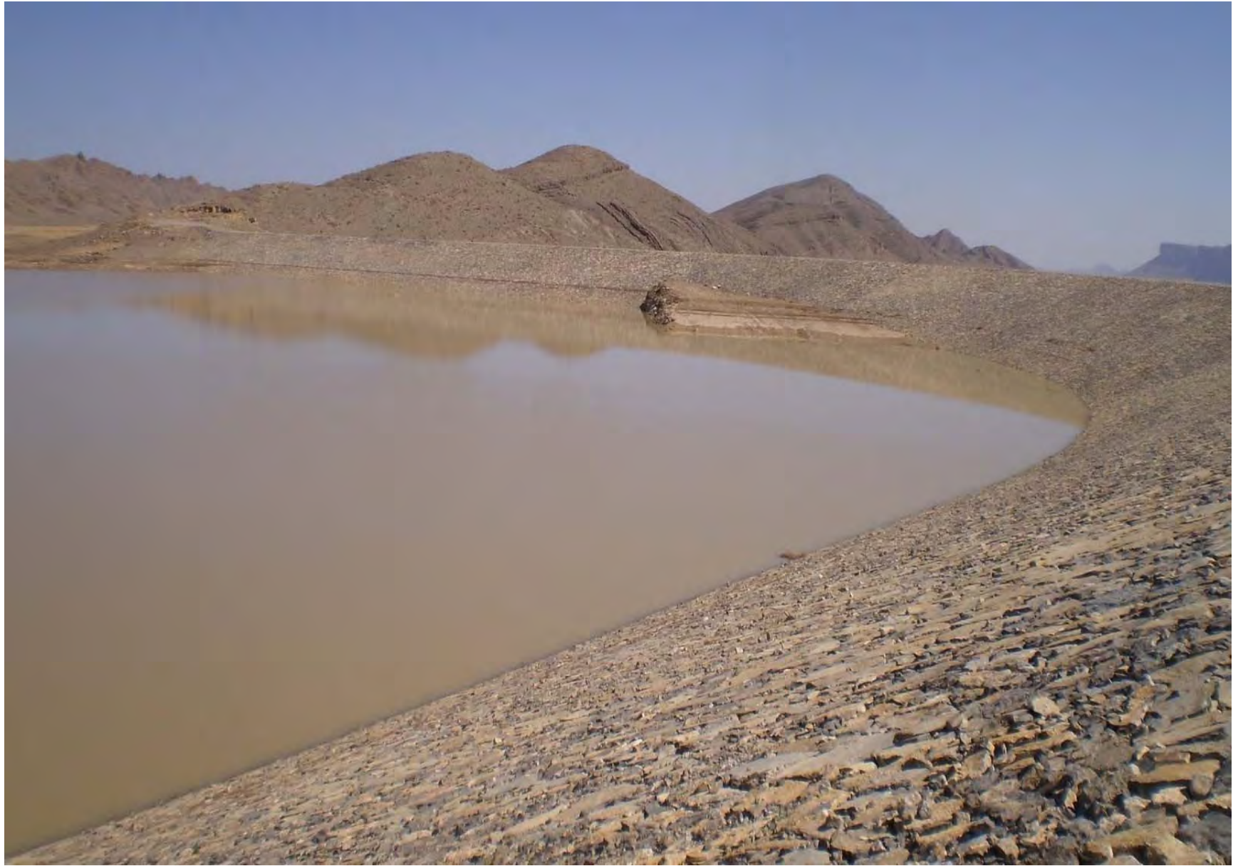
Surghund Dam - A View of Reservoir, District Loralai
