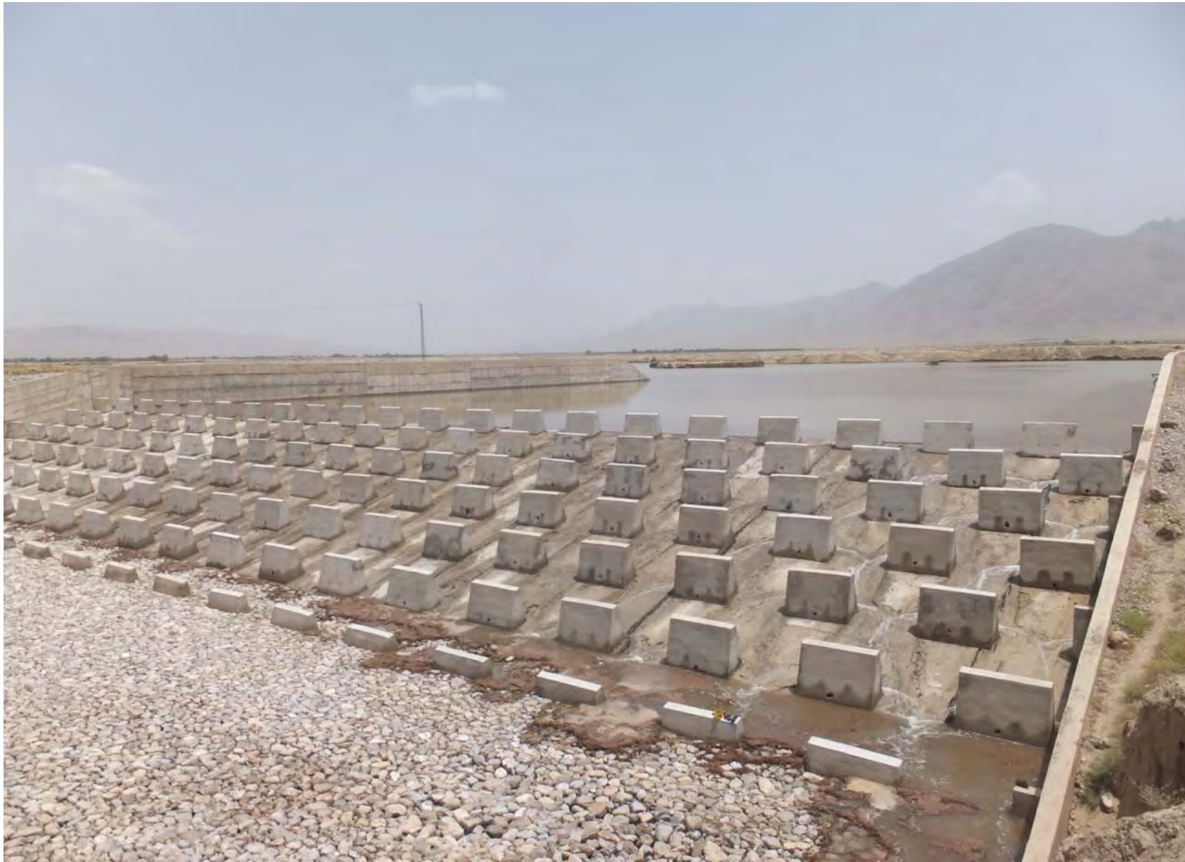
Bostan Dam – Distirct Pishin
