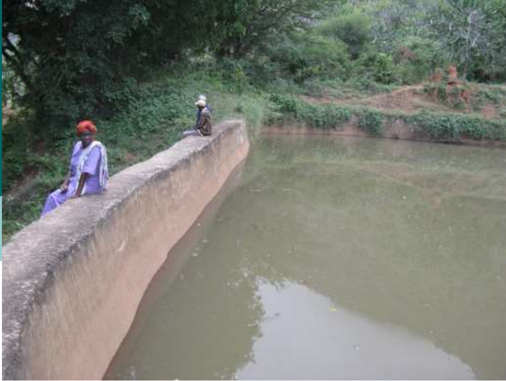
Microdam night storage structures
