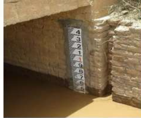
Installing gauge staff
