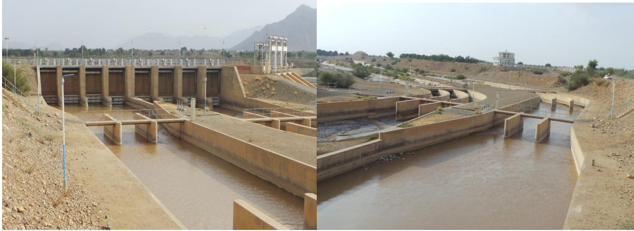
Figure 3. Main canal with its settling basin of the Wadi Mawr scheme
