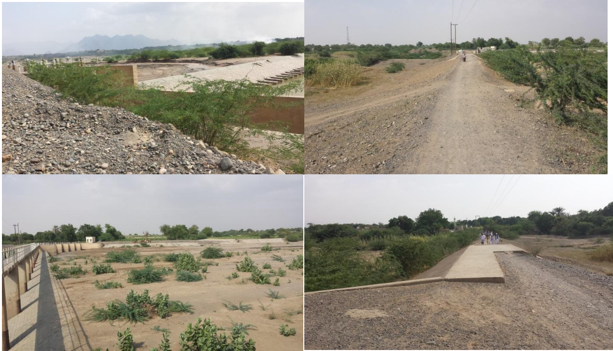
Figure 4. View of the Wadi Zabid spate irrigation weirs
