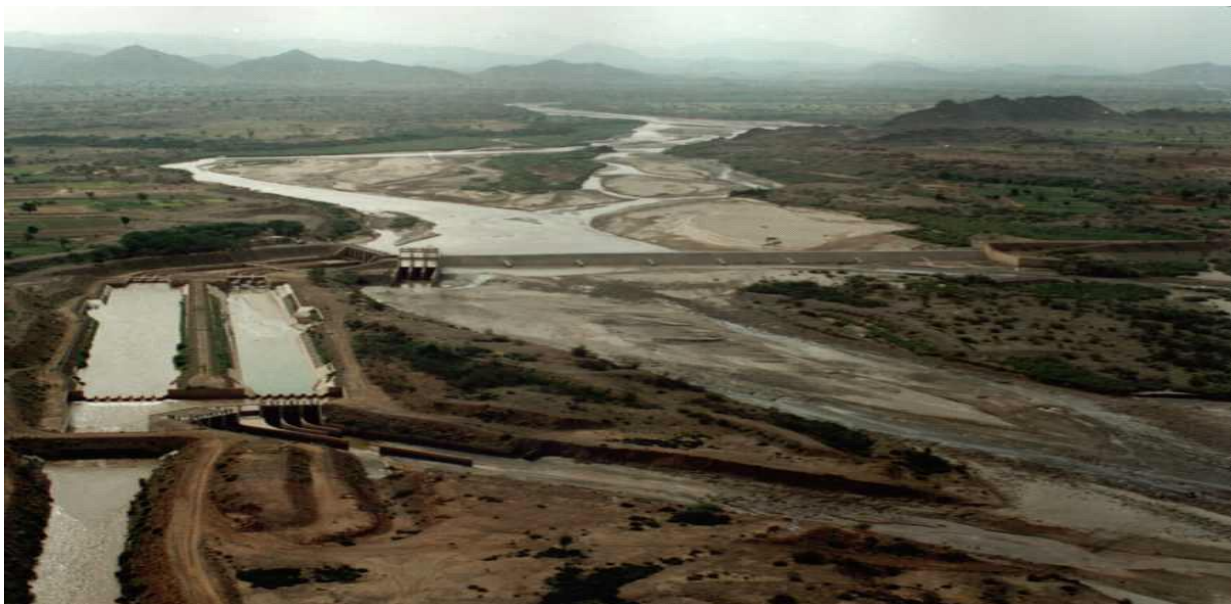
Figure 2. Overview of Wadi Mawr diversion structure
