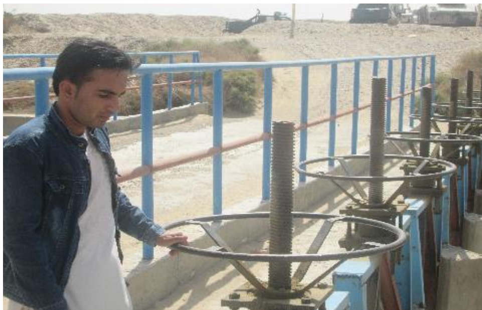
Figure 4; Regulator over Lashkari Canal for controlling flow of water during different seasons
