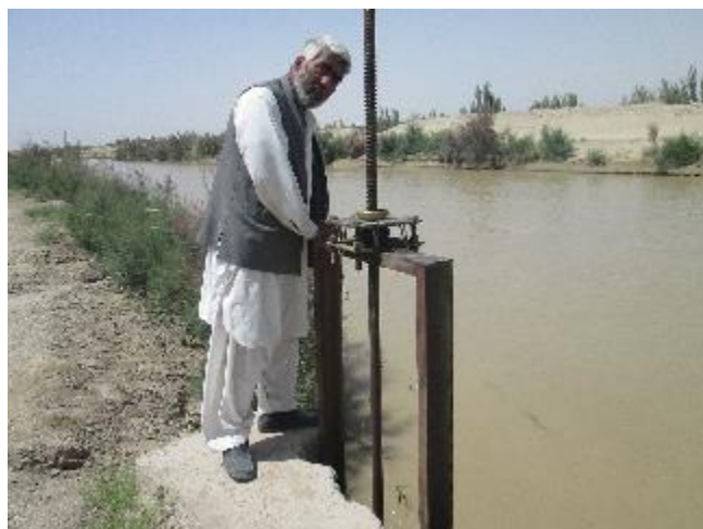
Figure 14; A control installed over Lashkari Canal for controlling flow of water to sub-canal; however the proprietor of jui welded the gate open to avoid its closing by mirabs to get more water than supposed to
