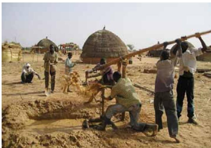
**FIGURE 3.3:** Washbore drilling
