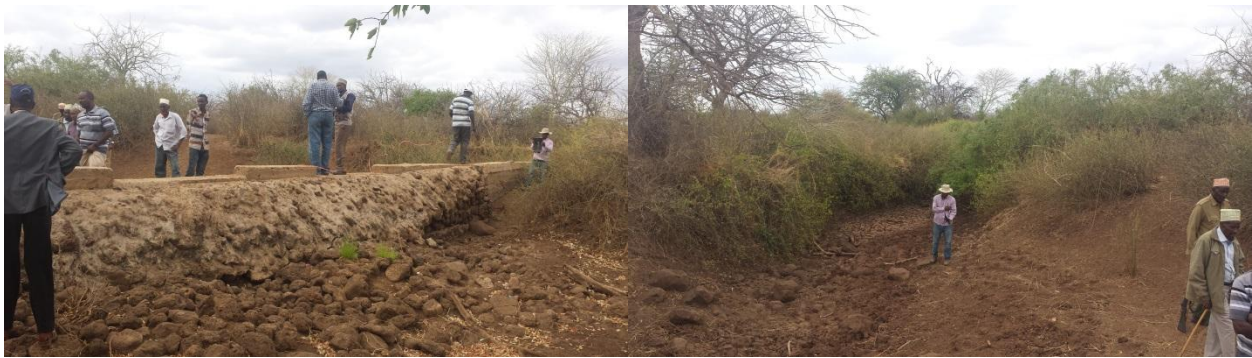
Figure 12 Existing check dam and the laga at its immediate downstream
