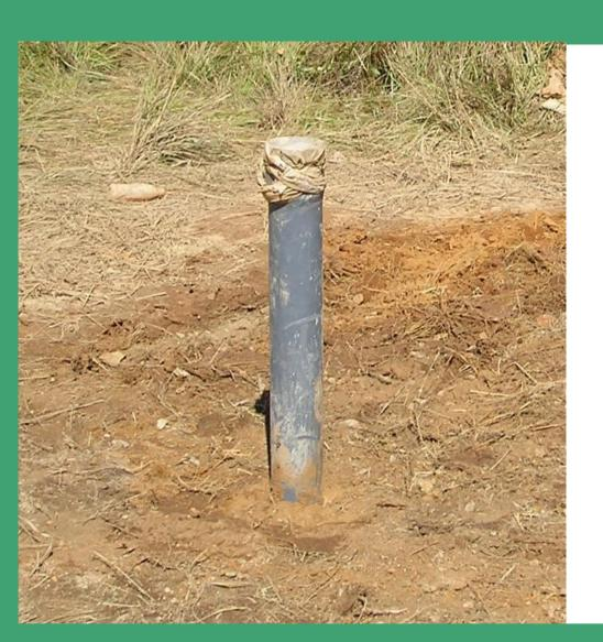
Manually drilled tube well
