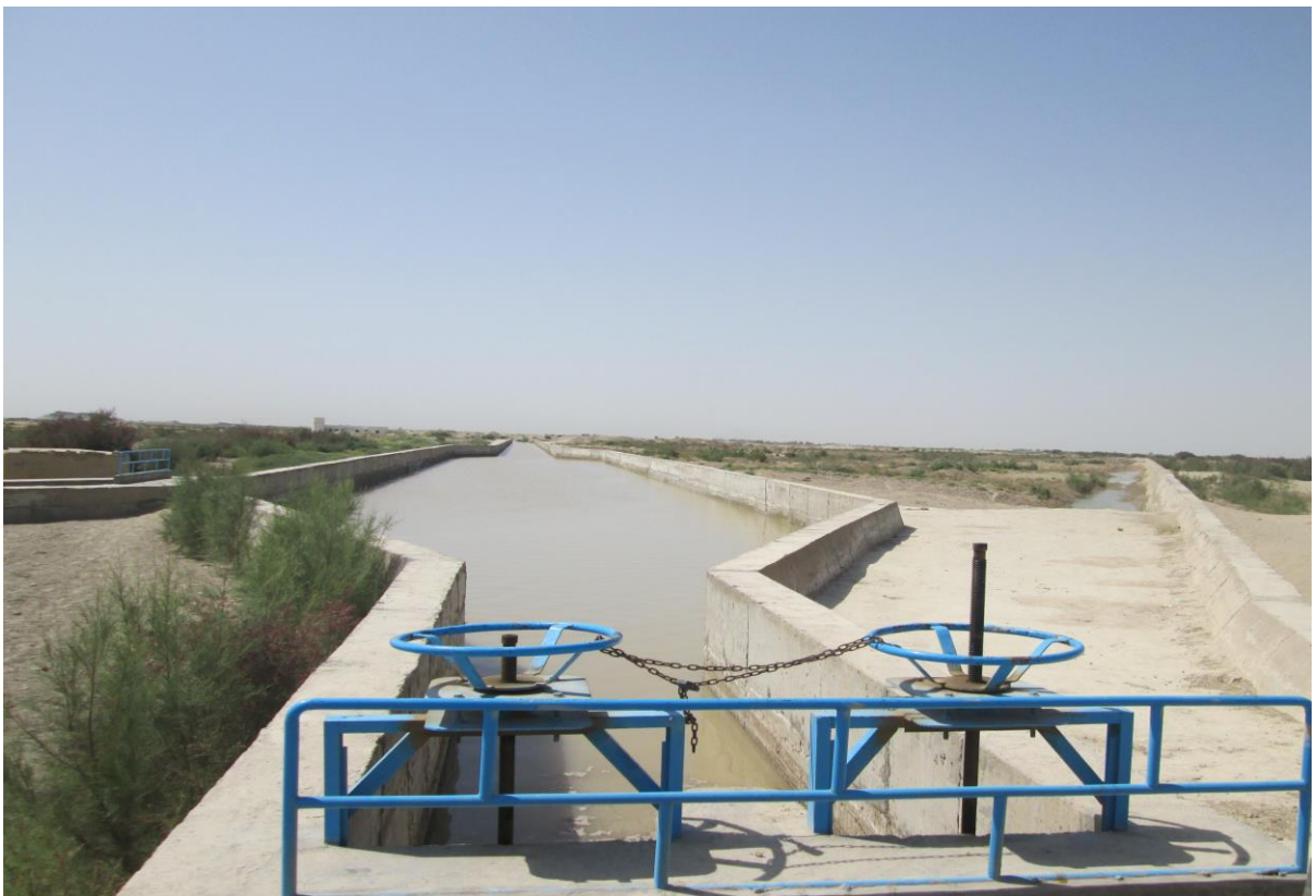
Figure 7: siphon at termination of Lashkari Canal which after that the canal joins Helmand River
