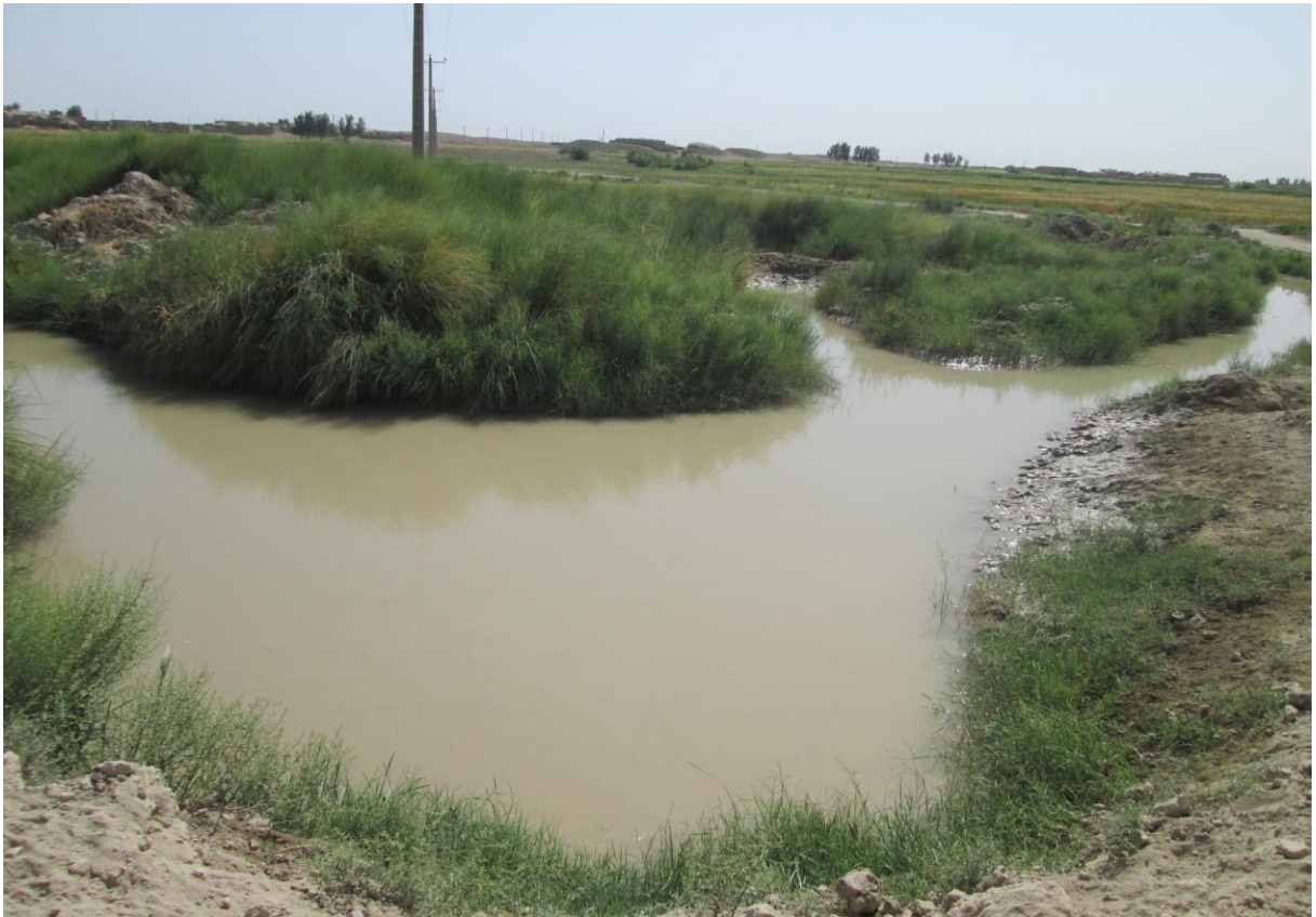
Figure 6: water sharing from a canal to sub-canals/juis (there is no control gate due farmers agreement in this level of water distribution)
