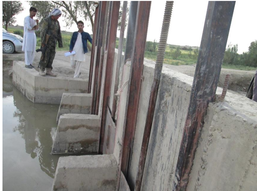
Figure 8: control gates over Lashkari Canal which some of them are broken by downstream users to allow water for downstream and also by upstream users to close them and to raise level of water
