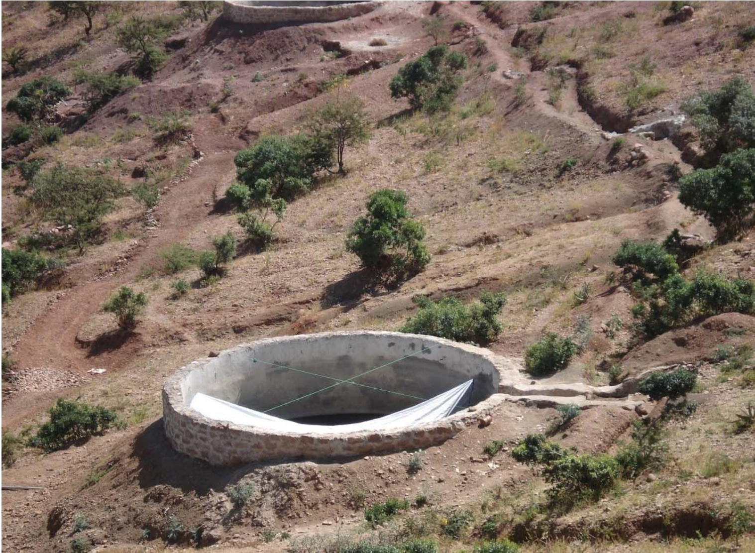
Series of underground tankers at Kola Tembhan Wereda
