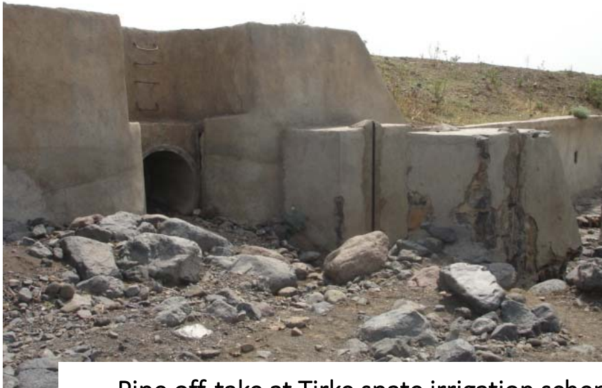
Pipe off-take at Tirke spate irrigation scheme before and after it was filled with sediment
