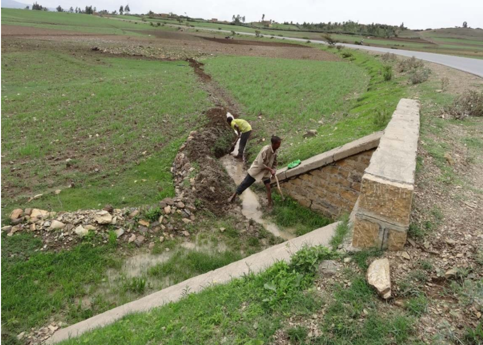
Road (a) and Culvert side Water Harvesting in Tigray Region
