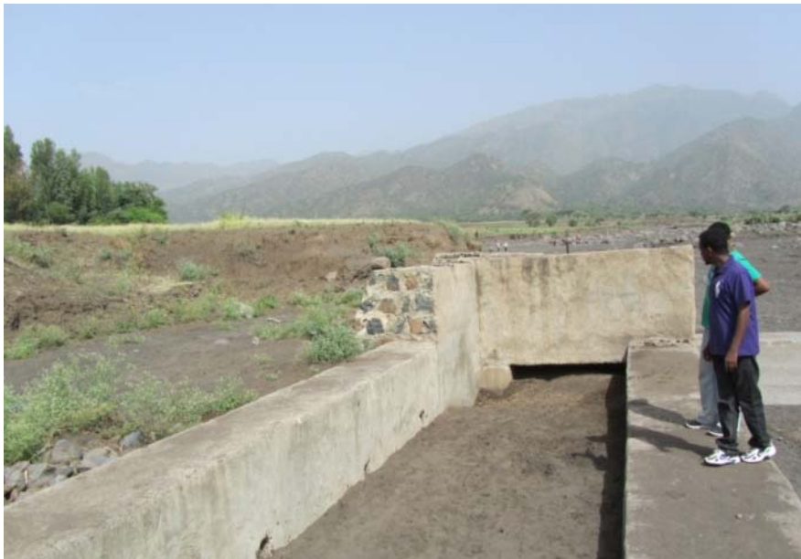
Box culvert off-take and siphon crossing at Hara spate irrigation scheme
