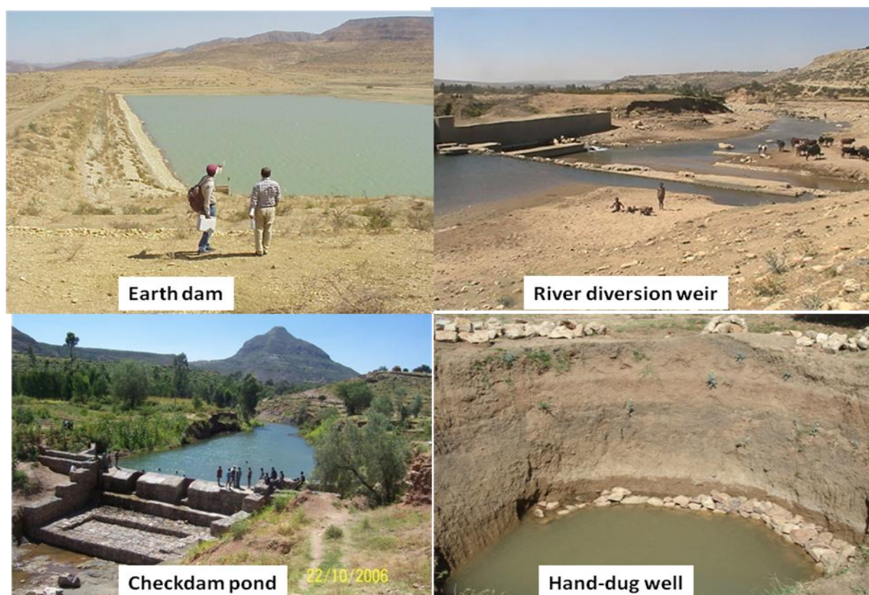
Figure 29 Some of the watershed management water harvesting techniques in Tigray in addition to FBFS
