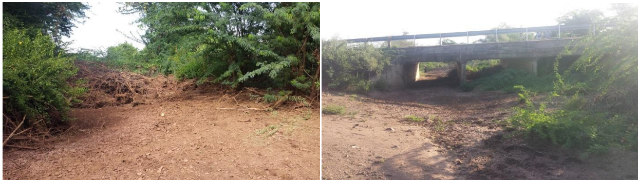
Figure 19 Flood diversion point and culver crossing at and upstream of Lomidat site
