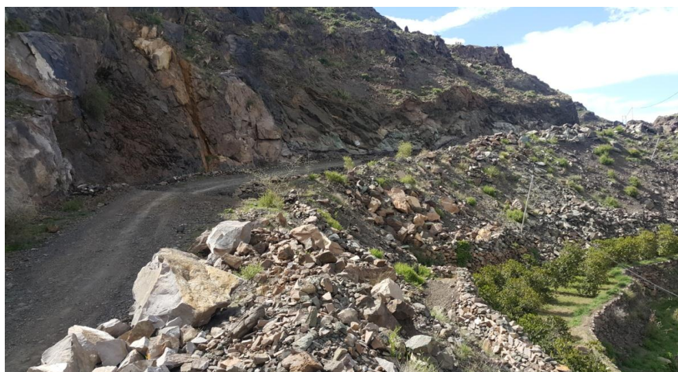
Figure 71 Road Rainwater Harvesting to Coffee Terraces using Earth Hump and Dry stone check walls.
