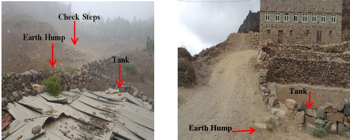
Figure 25 Right: Earth check steps to divert the surface runoff to the tank by earth hump, Left: Open water harvesting tank and an earth hump
