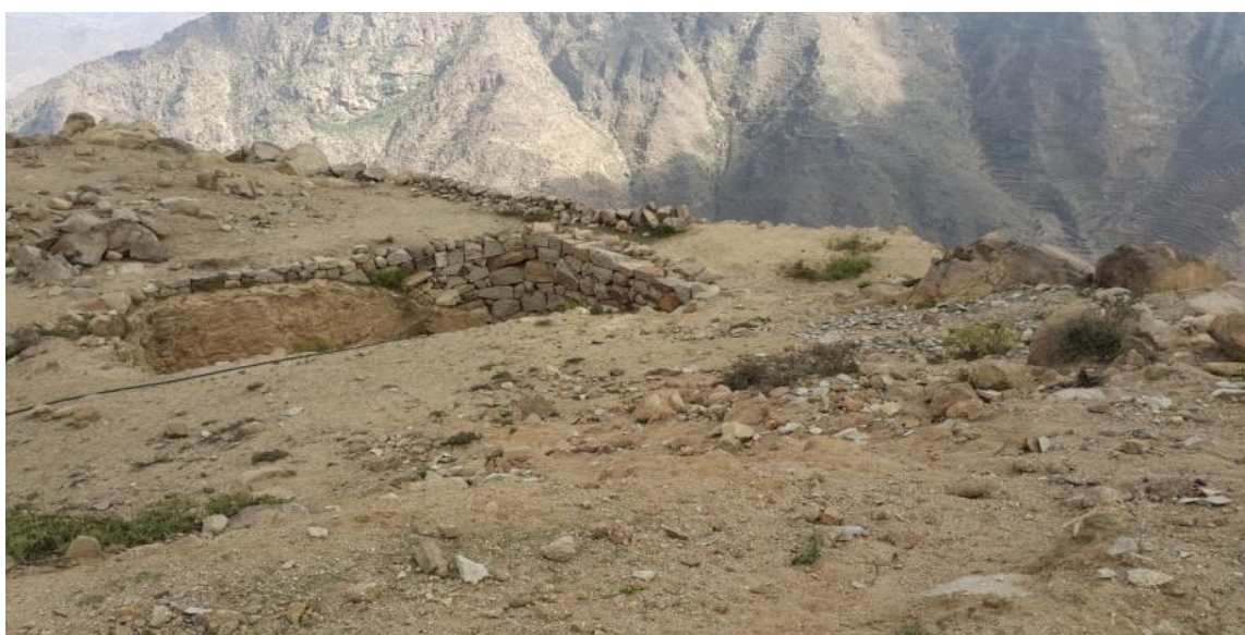
Figure 15 Under construction tank
