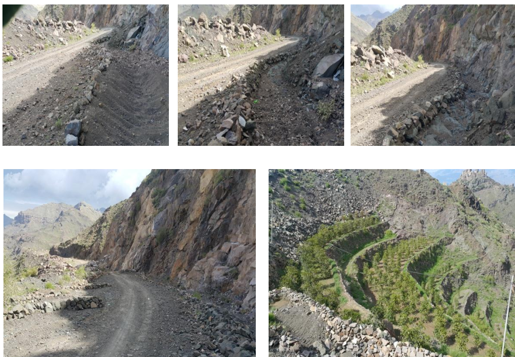
Figure 70 These photos show the farmer technique to harvest water across the road using dry stone check walls (along the road and skew)
