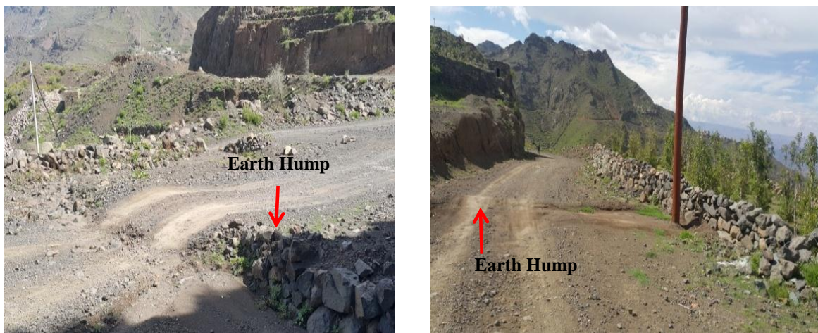
Figure 24 Earth humps to divert the surface runoff to the farms
