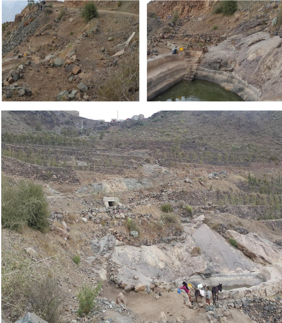
Figure 75 Water harvesting pond from culvert outlet
