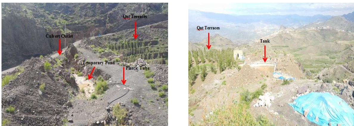
Figure 69 Water harvesting tank at the culvert outlet, (left picture) shows the temporary sedimentation and storage pond and the plastic tube to transfer the water to the harvesting tank (right picture)
