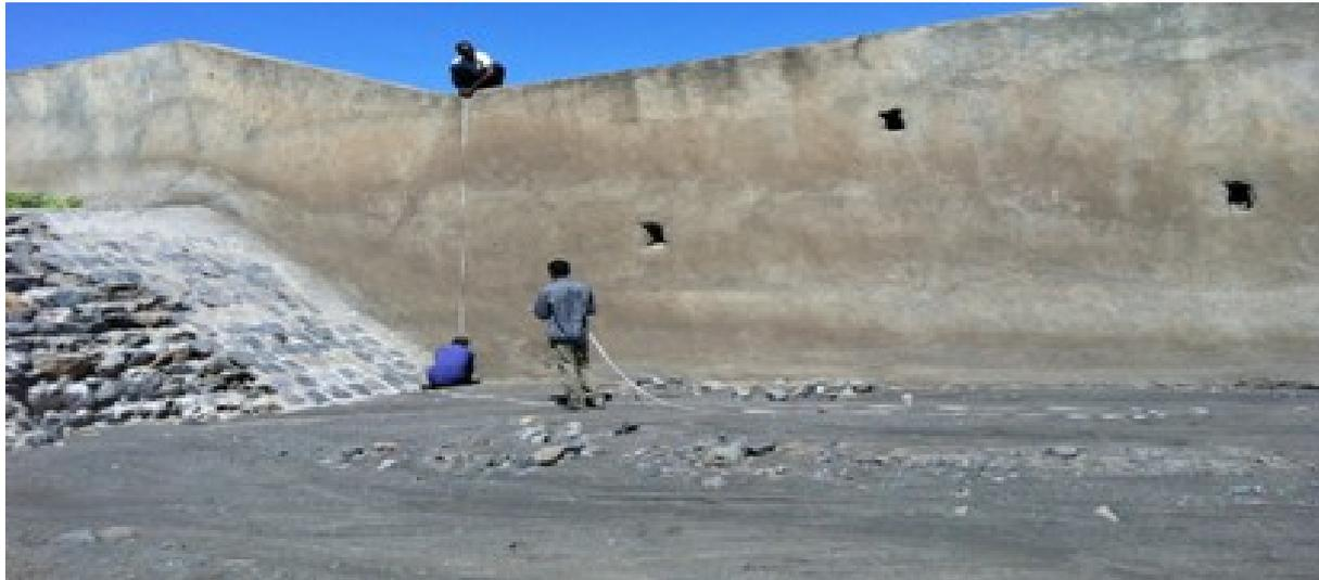
**Figure 4.3** Measurements of diversion structure dimensions in Dayu scheme
