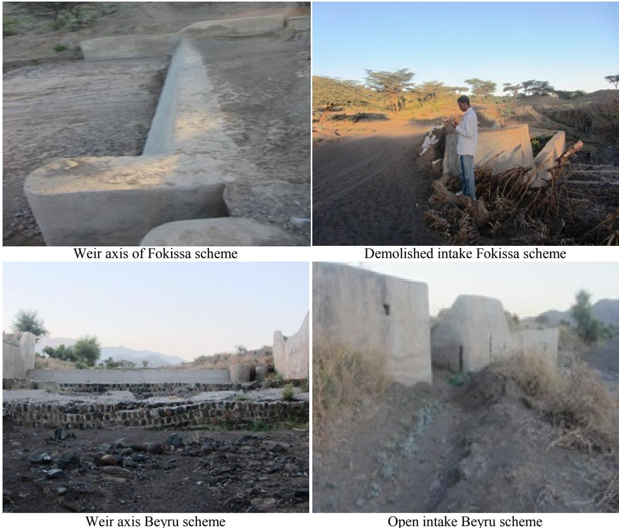
**Figure 6.2** Headwork structures of Fokissa and Beyru spate schemes
