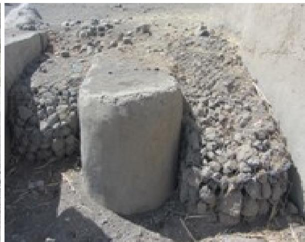
Sluice gate blocked by gabion, Tengago
