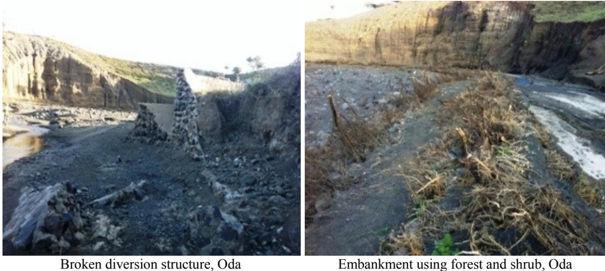
**Figure 6.4** headwork structure of Oda spate irrigation system
