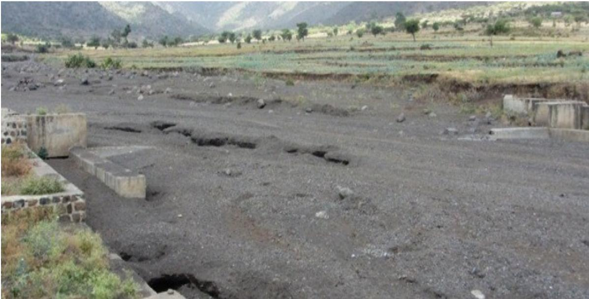
**Figure 1.3** Unsuccessful modernized spate irrigation scheme in Hara, Raya valley
