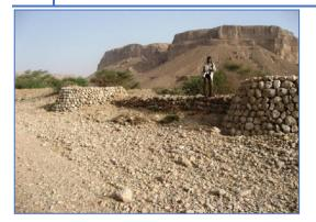
Controlled overflow structures help water getting from a fully filled field to the next in a controlled way – avoiding breaching of the side bunds and gullying and rutting from the water that rushes out of the field. There are several examples of such controlled overflow structures (orifice with a silting basin,).
