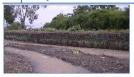
Construct channels to guide spate water within the field and between fields.
