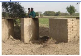
When a large bunded field is filled with floodwater, it is a challenge to prevent the water rushing back. Field closure gates can be constructed to control the flow and avoid erosion in field to field systems.
