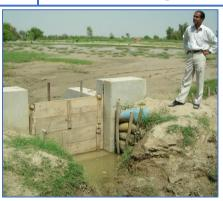
It is important that a field is drained properly and does not have standing water. Make simple structures to remove excess water from the field to reduce or eliminate water logging and return soils to their natural field capacity. Examples are subsurface tile drainage systems, surface disposal drains and two and three-tier drainage systems.
