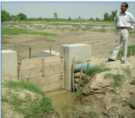
*It is important that a field is drained properly and does not have standing water. Make simple structures to remove excess water from the field to reduce or eliminate water logging and return soils to their natural field capacity. Examples are subsurface tile drainage systems, surface disposal drains and two and three-tier drainage systems.*
