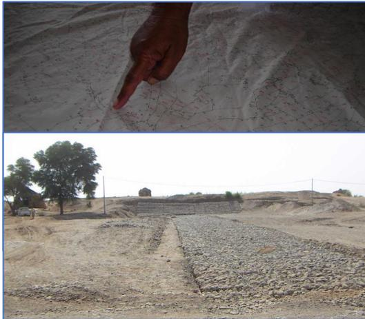
*Discuss how to fairly share the water within the command areas and in such a way that it is efficiently used (clear and transparent rules and arrangements) – looking at making (1) bed stabilizers at distribution points (2) permeant flow dividers (made of gabion) (3) bed raisers.*
