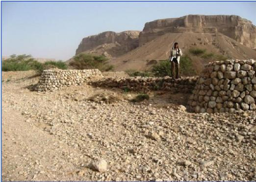
Controlled overflow structures help water getting from a fully filled field to the next in a controlled way – avoiding breaching of the side bunds and gulying and rutting from the water that rushes out of the field. There are several examples of such controlled overflow structures (orifice with a silting basin,).
