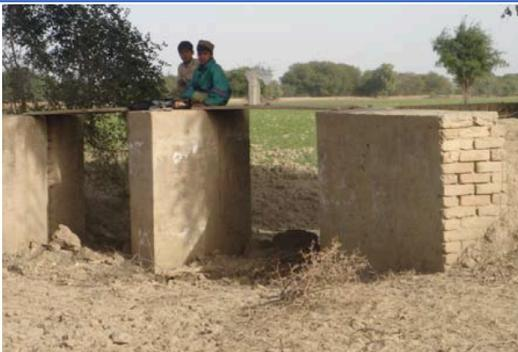
When a large banded field is filled with floodwater, it is a challenge to prevent the water rushing back. Field closure gates can be constructed to control the flow and avoid erosion in field to field systems.
