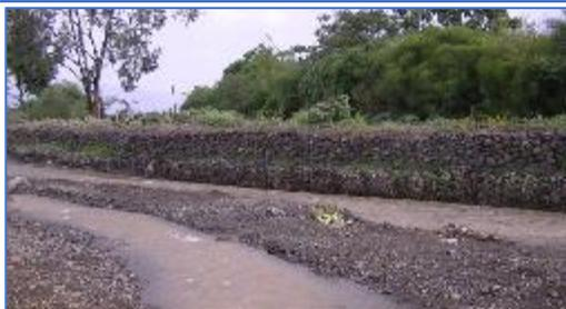
*Construct channels to guide spate water within the field and between fields.*
