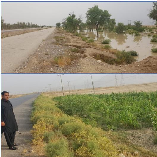
*Harvesting run-off water from roads by using channels and culverts and spread this over land to provide additional water for crops/grasses/trees, collect it in storage structures (like roadside ponds, small depressions turned in oasis) or spread it over areas with high infiltration to boost shallow aquifer recharge.*
