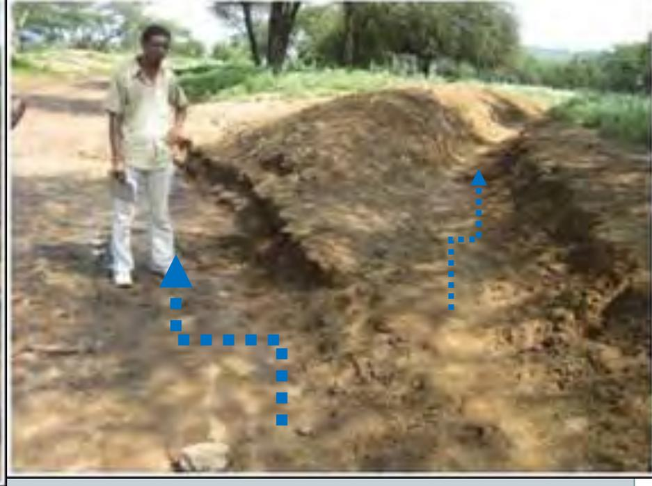
Figure : Lowering of the bed of branch channel, by farmers, to irrigate the field at head that was lost due to sedimentation, Luka Kebele – South Omo , Ethiopia
