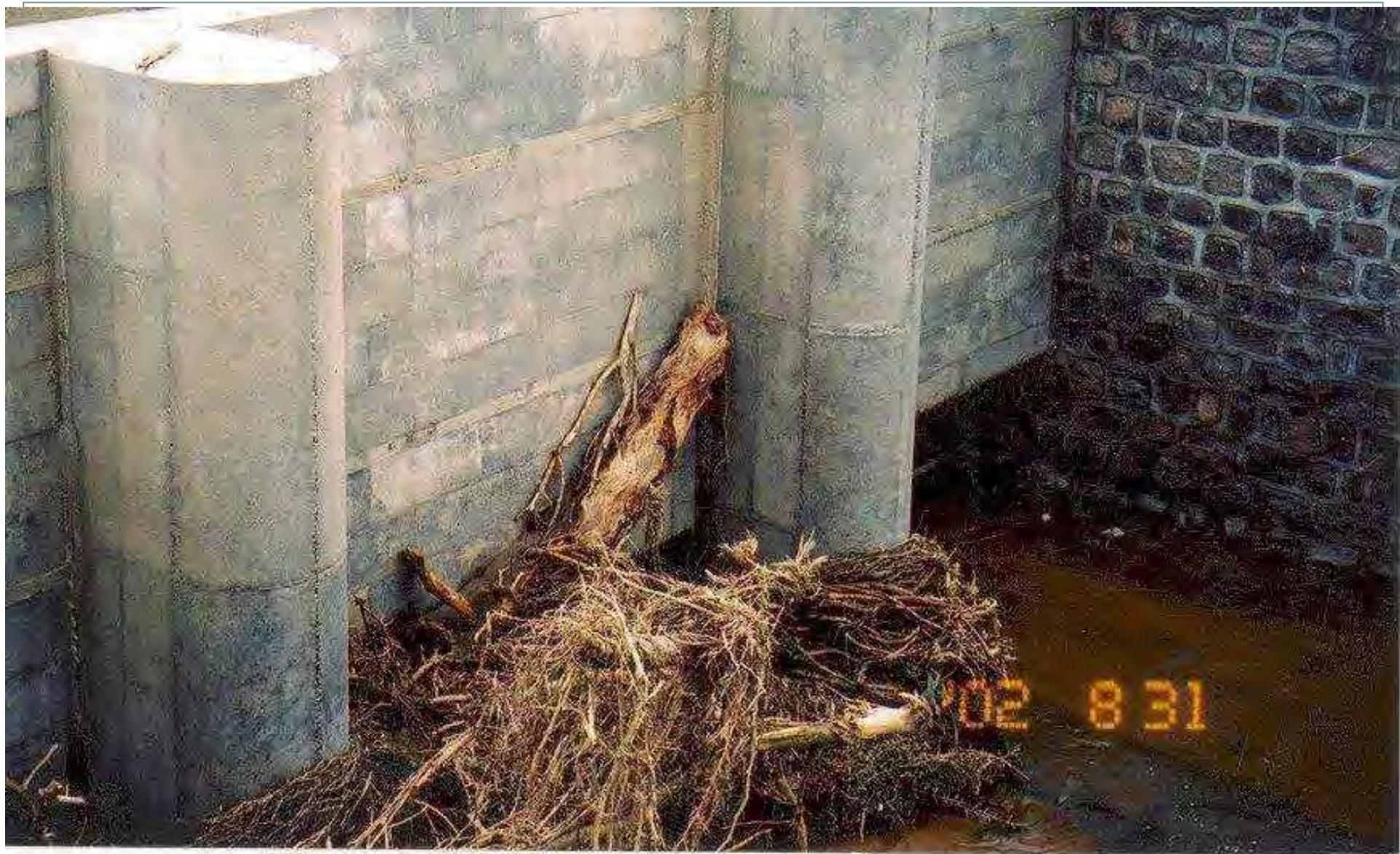
**Figure: Short coming of the so far modernized structures: Trash transport / blockage**
