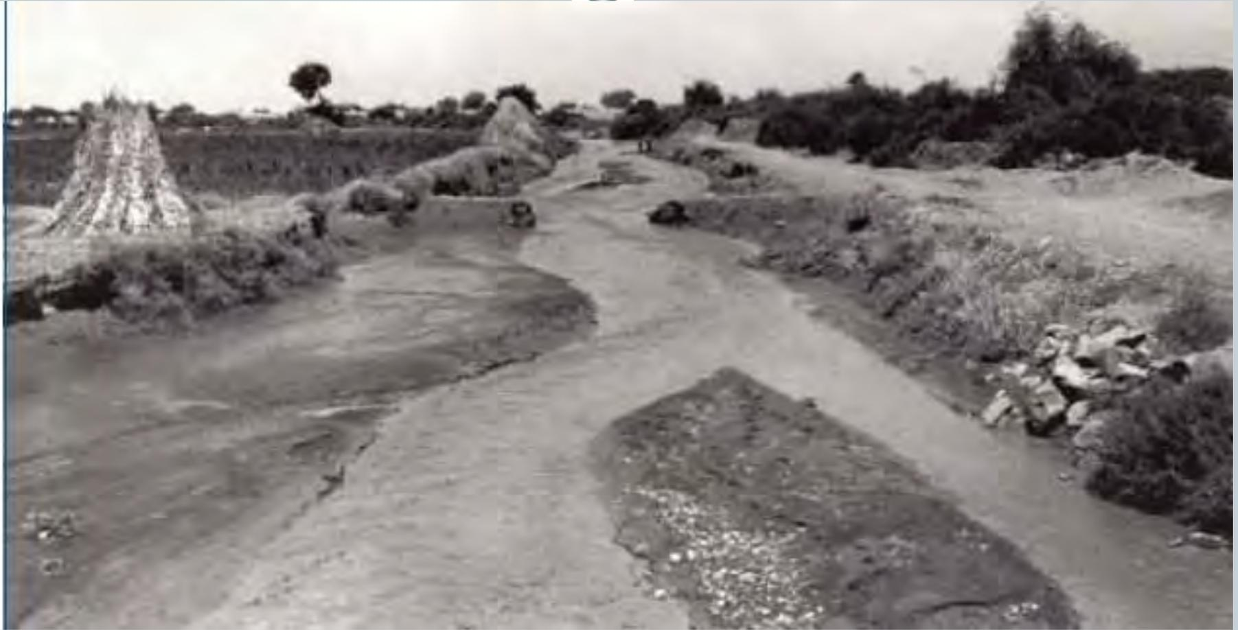
Figure: Traditional flood diversion: spur-type deflector
