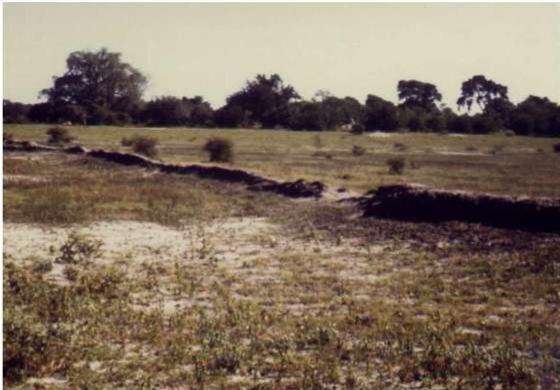
Figure 2.5. An old, abandoned bund made to retain water in the *molapo* (from: Oosterbaan et al., 1986).
