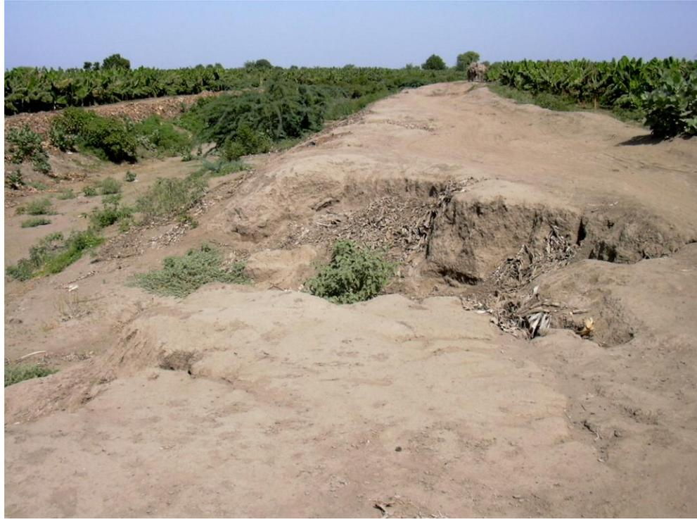
*Deep Incised Cut in Mansuri Canal Bank Due to Flooding*
