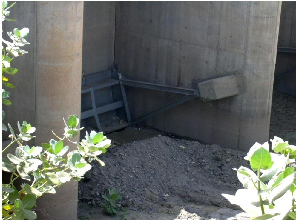
*Deposited Sediment In Front of Head Regulator*
