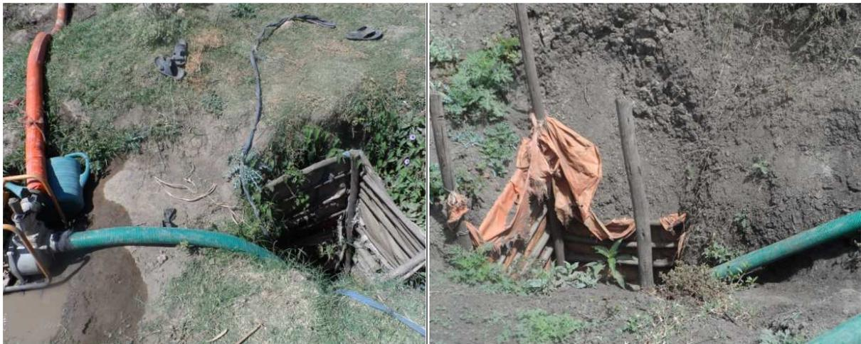
**Figure 5.17** Hand-dug wells with protection material
