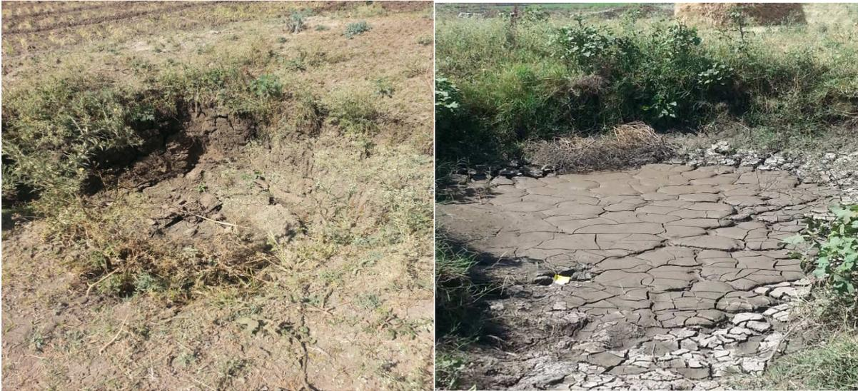
**Figure 5.13** Collapsing and sediment deposition of hand-dug wells
