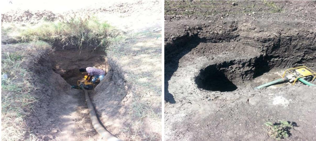
**Figure 5.14** Pump position relative to ground surface
