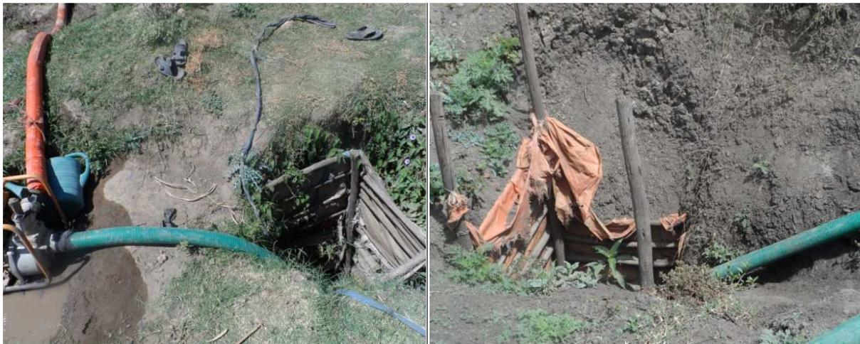
**Figure 5.17** Hand-dug wells with protection material
