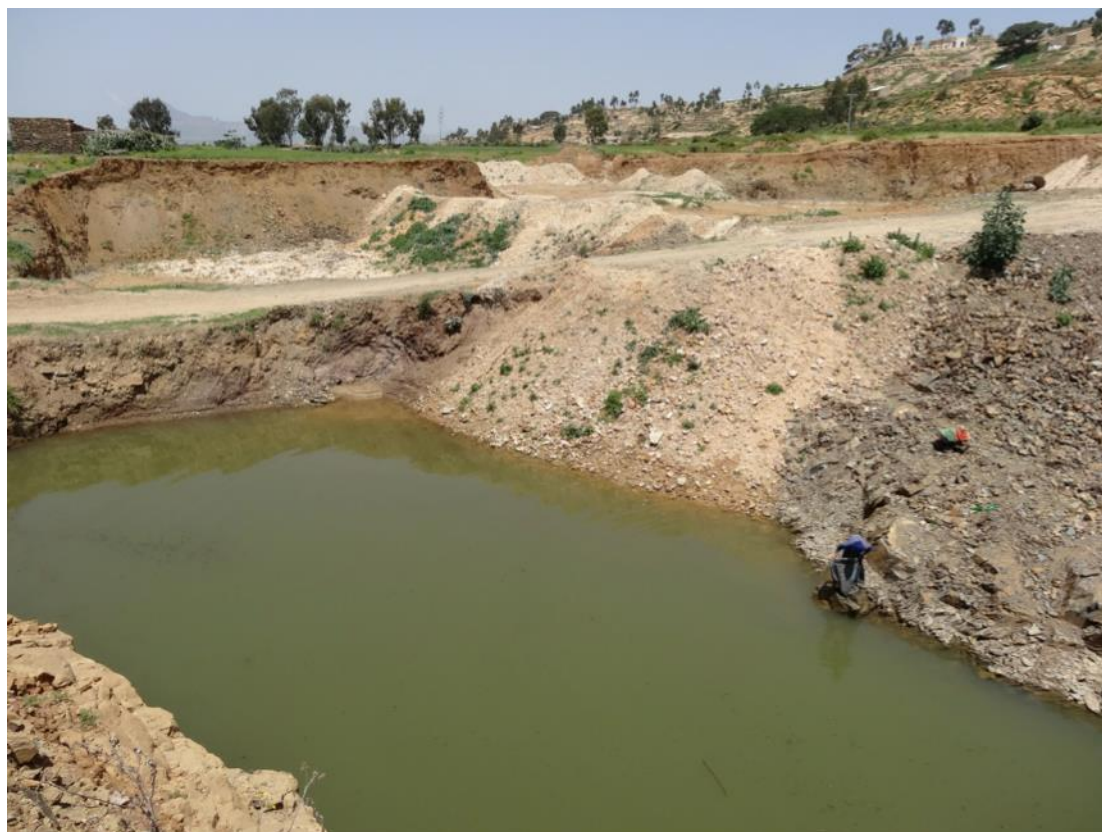
Figure 2: Borrow pit collecting and storing surface runoff in Tigray region, Ethiopia. Photo: MetaMeta.
