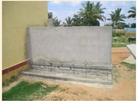
Water taps outlet system and cemented area below the tap for letting wastewater disposal
