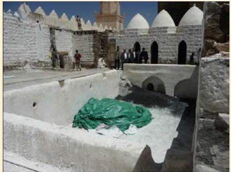
Roof rainwater harvesting from a Mosque roof to mousque pond in Jiblah, Yemen (poho: sharaf 2011)
