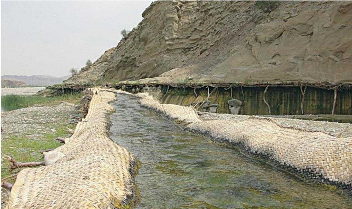
spread and bended. Nai water pressure is used to push water climb on this manual made water course and this water through *mad* irrigation is used to irrigate the lands at upper places.
